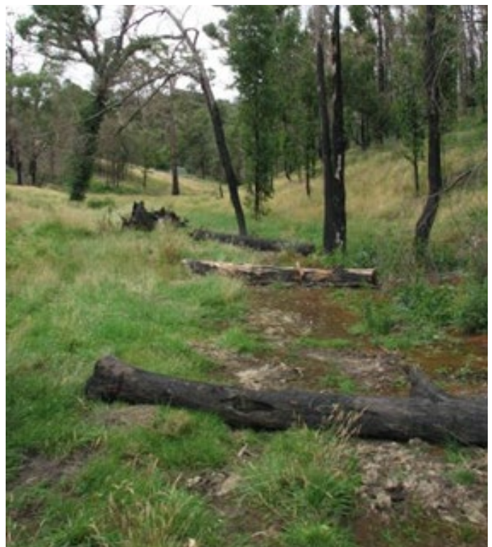
Plate 19 Log check dam from trees in burnt area
