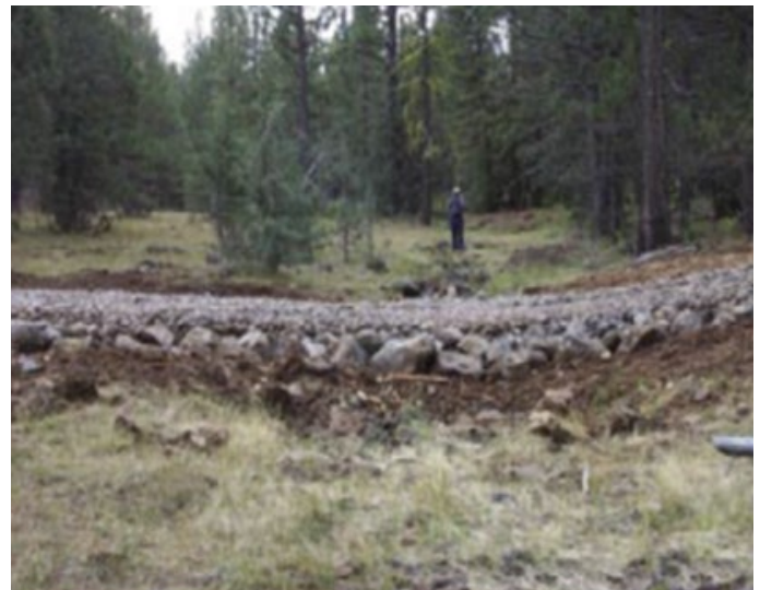
Plate 23 Armoured Rolling dip (USDA 2006)
