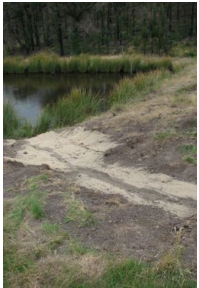
Plate 15 Fibre blanket near waterway where sheet erosion may occur
