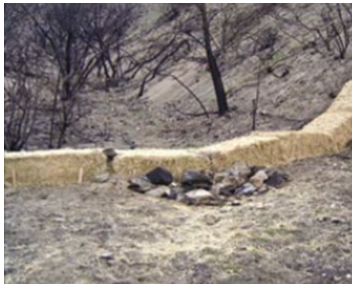
Plate 18 Strawbale check dam with energy dissipater (USDA 2006)
