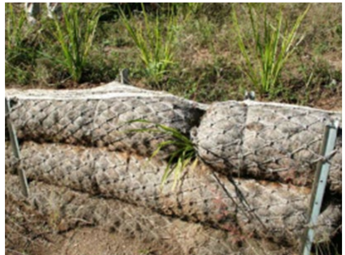
Plate 22 Terraced geo logs (IECA 2010)
