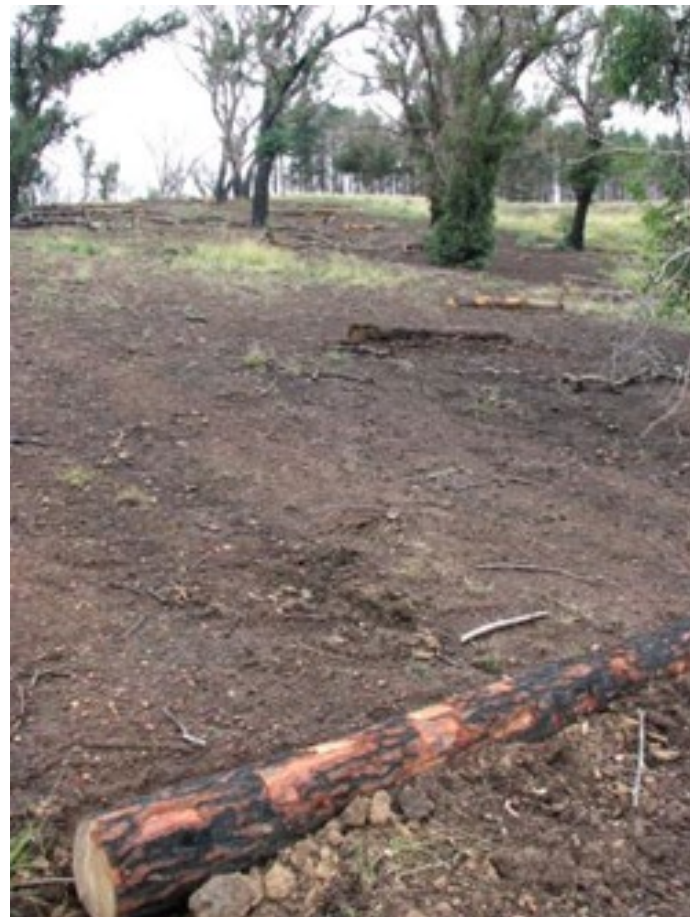
Plate 17 Log erosion barriers on severely burnt slope
