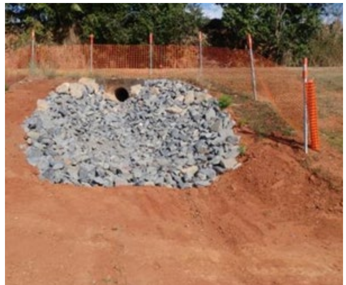
Plate 24 Rock lined overside drain (Roberts 2017)
