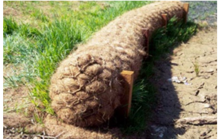
Plate 21 Geo log placement in a single line (IECA 2010)
