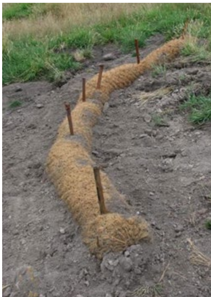
Plate 16 Fibre roll on slope where erosion control is required
