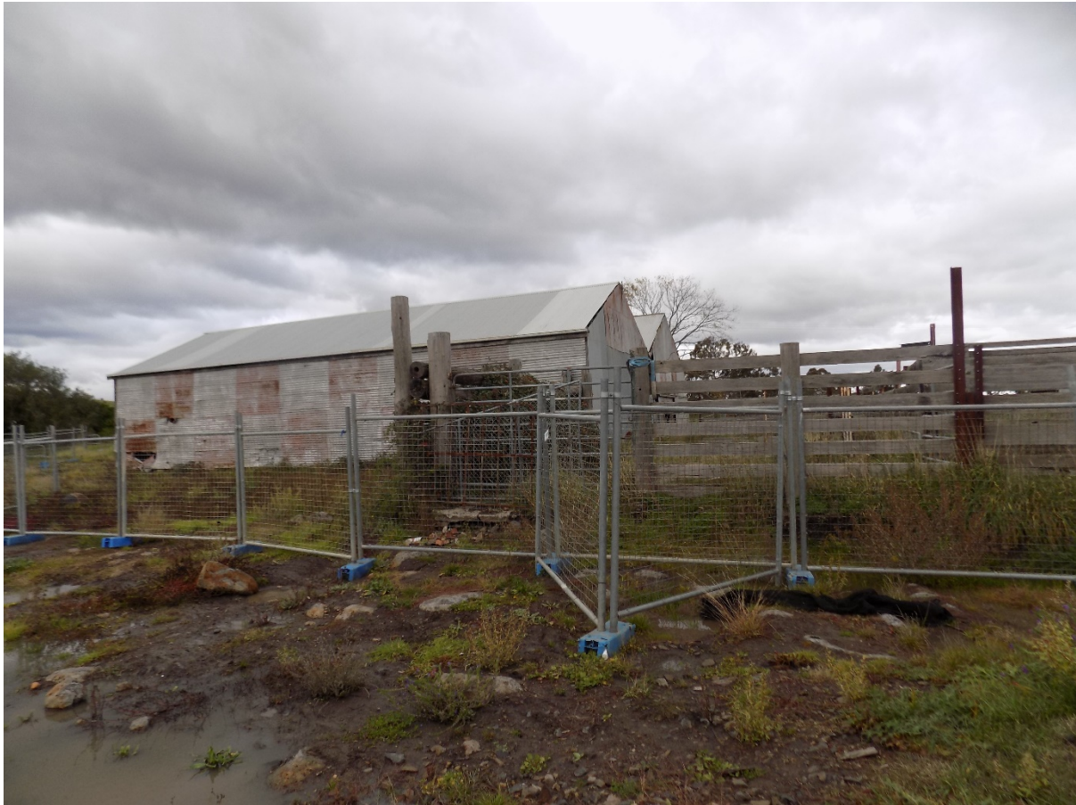
Figure 14 – South southeast from east end of 130 Bindts Road driveway. 20 May 2020.
