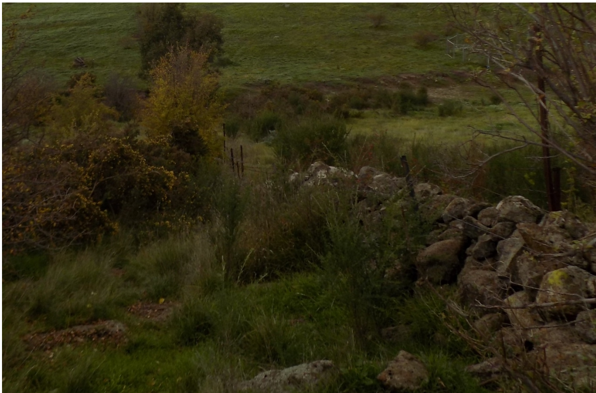
Figure 23 – East along wall at boundary between 130 and 100 Bindts Road from junction with north-south dry-stone wall. Section is in path of Boulevard Connector Road required according to the Quarry Hills Precinct Structure Plan. 20 May 2020.
