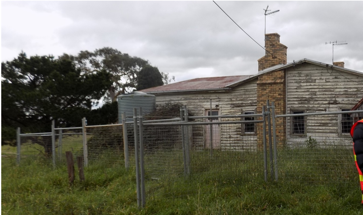
Figure 6 – North from the south side of the McKie dwelling. 20 May 2020. Shows external tank and lavatory
