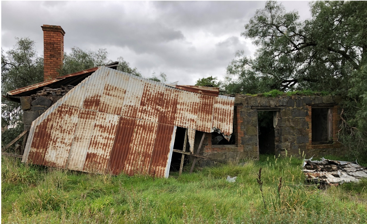
Figure 21 – North from south side of stone dwelling. 20 May 2020.
