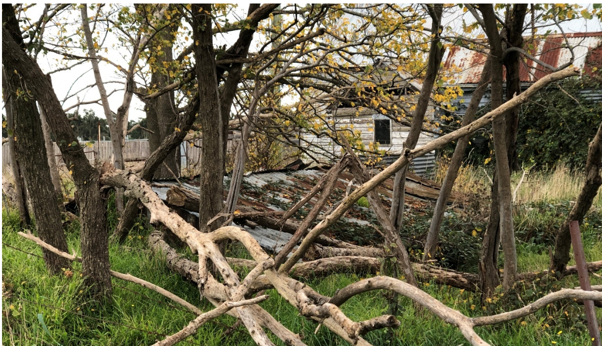
Figure 17 – North towards roofed well tank and other outbuildings beyond.
