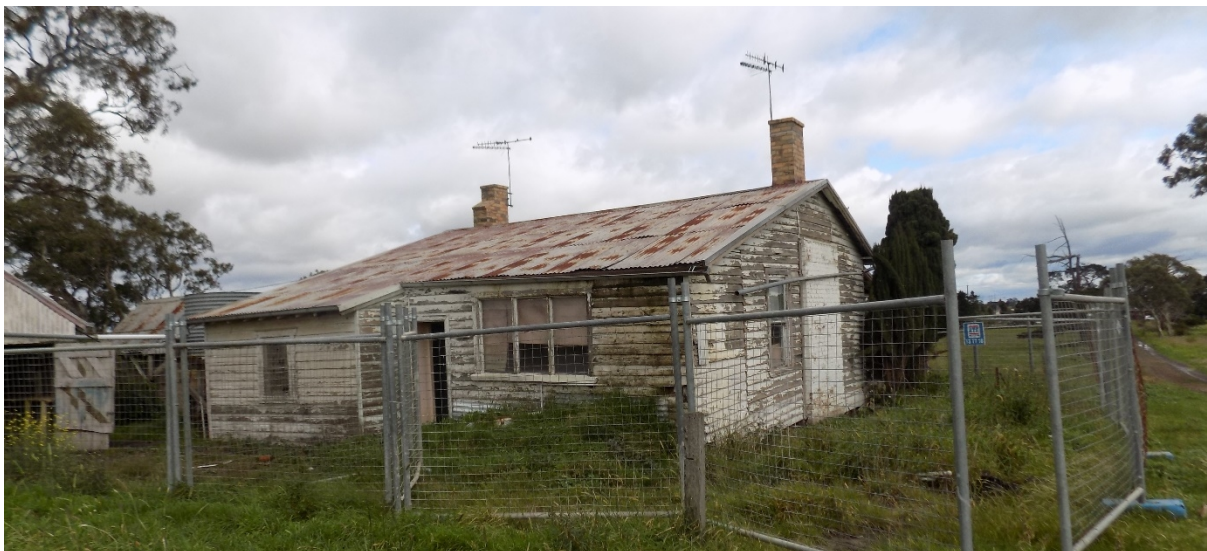
Figure 5 – West from the east side of the weatherboard dwelling. 20 May 2020
