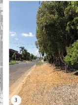
3 Informal footpath along the northern side of Boronia Street
