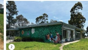
2 Sense of discomfort due to the lack of buffer distance between community centre and footpath
