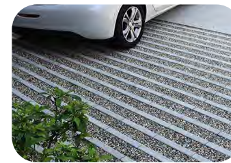
PERMEABLE CAR PARK
