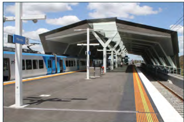
FIGURE 13- MERNDA STATION PLATFORM
