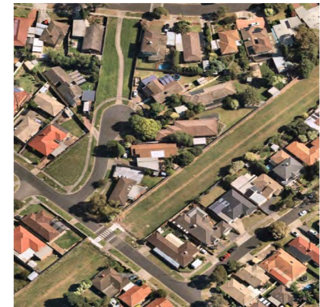
Figure 52 Image of easements passing through Mill Park with 1.8m rear or side fencing
