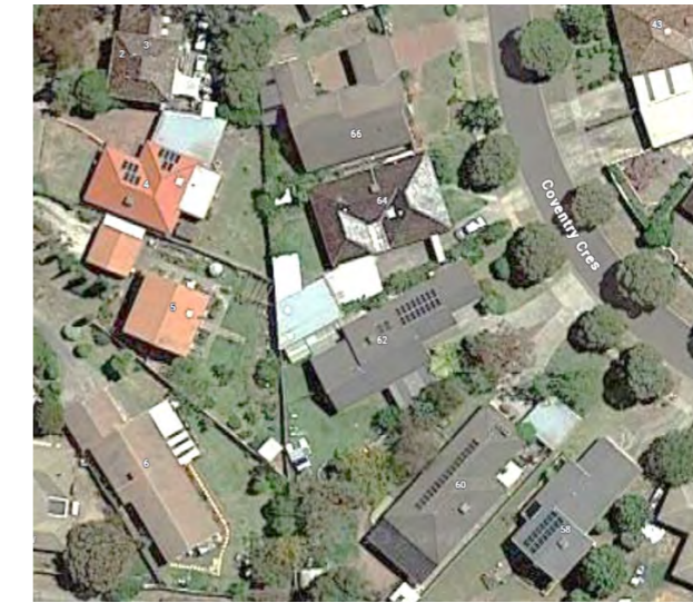
Figure 76 Gaps between buildings
