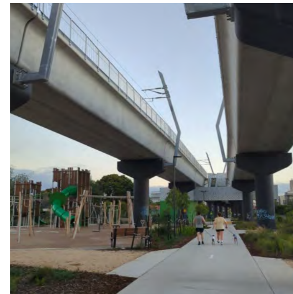
Figure 26 Linear park playground under elevated rail corridor between Bell and Preston station
