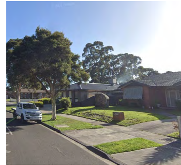
Figure 74 Low, single storey
