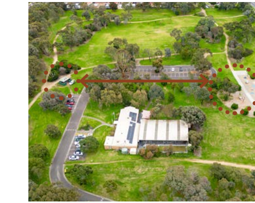
A The toilet is situated at a distance from the playground
