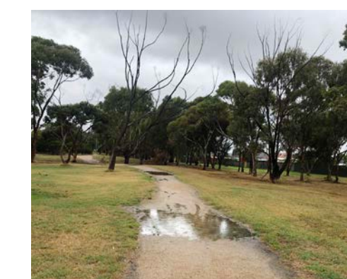
E Pathway areas are subject water logging in wet weather
