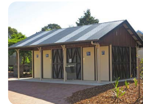
Example of toilet facilities
