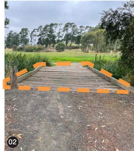
02 Existing bridges - in poor condition and not DDA compliant
