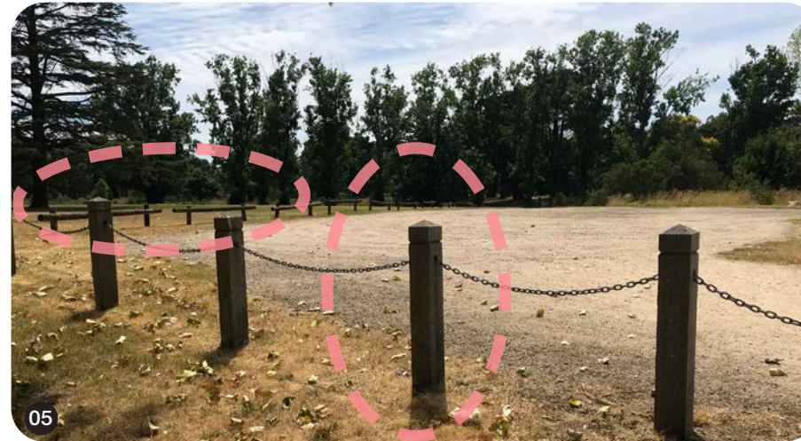
05 Example of vehicle exclusion barriers throughout the site
