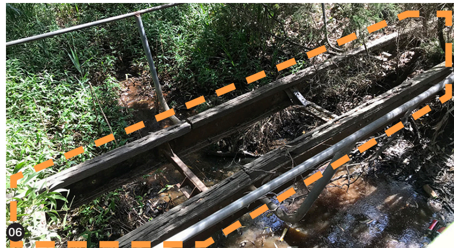
06 Example of outdated structures remaining alongside new bridges, assess for historic value and remove or protect
