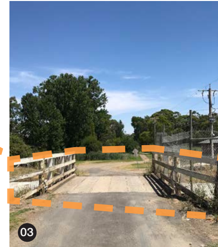
02 Existing bridges - in poor condition and not DDA compliant
