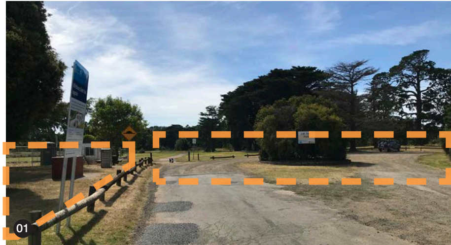
01 Walnut Street arrival point, with informal parking area, vehicle exclusion barriers and BBQ picnic area (not DDA compliant)
