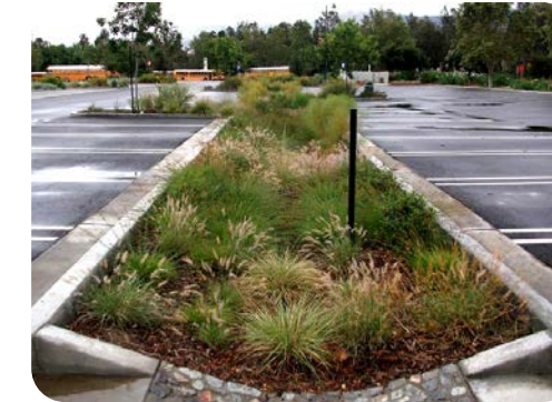
Example of carpark raingarden
