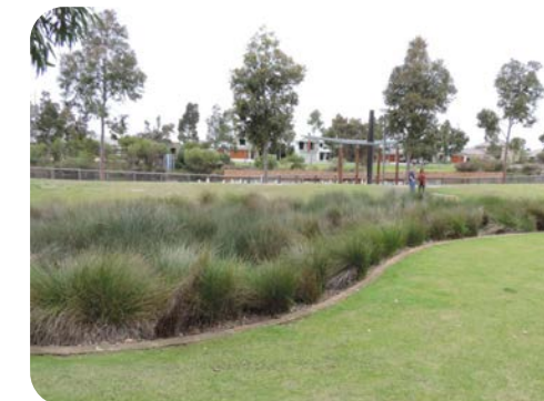
Example of planted drainage swale
