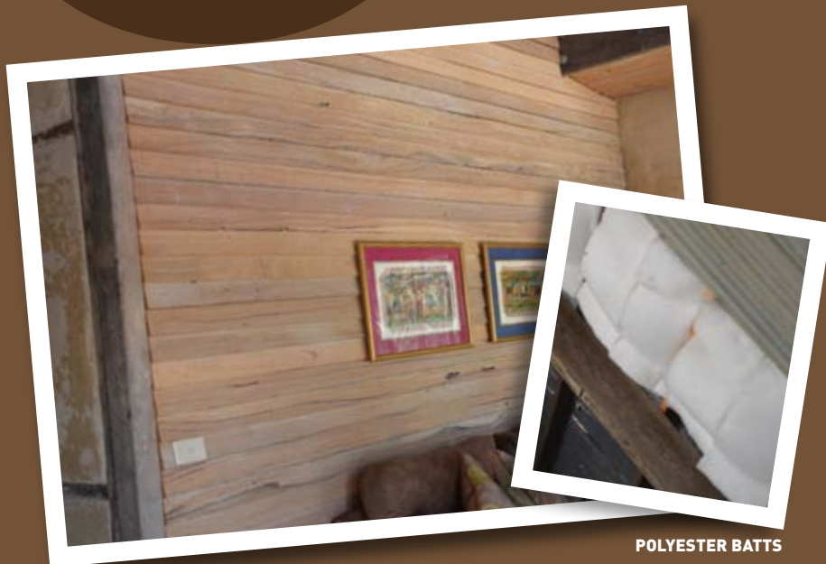
RECYCLED TIMBER WALL
