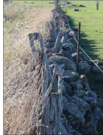
Images 137, 138: Part of the western boundary of 80 Harvest Home Road with the former Unmack family at 90 Harvest Home road, comprises the substantial remains of a rare composite stone, post & rail, post & wire wall, as described in a 1968 survey, and photographed in 2011 (left), and 2019 (right). Robert Wuchatsch remembers many composite walls in the area, but examples with very old heavily mortised posts are now rare. In 1990 Gould (Site 1.25) reported a 'post & rail' fence on the property, which may have been this one. The wide base would suggest that the posts may have been inserted sometime after an original all-stone wall was built, but other evidence, including some massive 'coping' stones suggest that it was originally a purpose-built half-wall. Further investigation of the fabric of the wall is warranted. (David Moloney, 2011, 2019)
