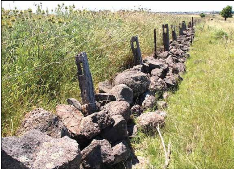
Images 137, 138: Part of the western boundary of 80 Harvest Home Road with the former Unmack family at 90 Harvest Home road, comprises the substantial remains of a rare composite stone, post & rail, post & wire wall, as described in a 1968 survey, and photographed in 2011 (left), and 2019 (right). Robert Wuchatsch remembers many composite walls in the area, but examples with very old heavily mortised posts are now rare. In 1990 Gould (Site 1.25) reported a 'post & rail' fence on the property, which may have been this one. The wide base would suggest that the posts may have been inserted sometime after an original all-stone wall was built, but other evidence, including some massive 'coping' stones suggest that it was originally a purpose-built half-wall. Further investigation of the fabric of the wall is warranted. (David Moloney, 2011, 2019)
