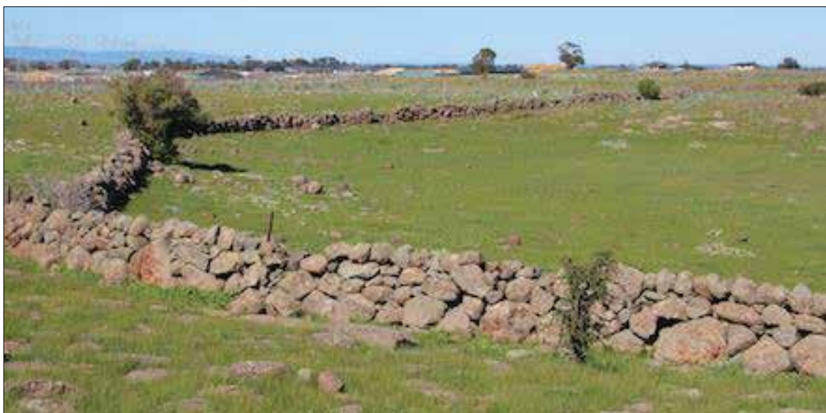
Image 22: A typical Merri-Darebin Plains wall, built along the top of a stony rise, separating grazing and arable land. The foundation level of the wall contains many oversize and massive boulders. Most copestones remain. (David Moloney, 2019)
