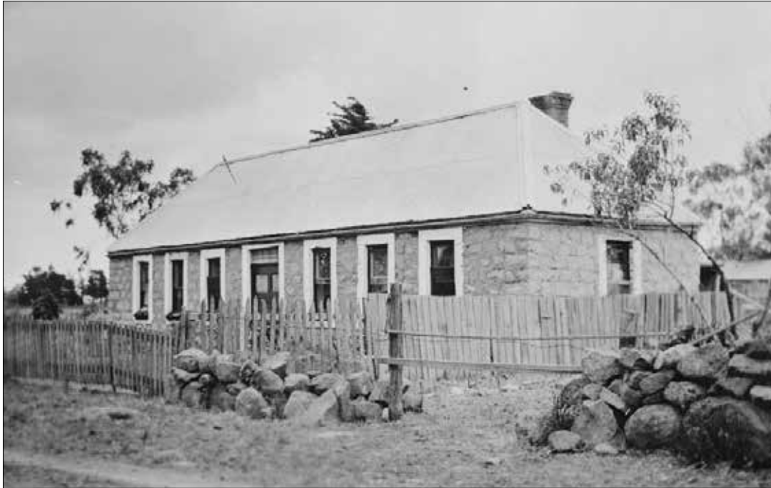
Image 109: By 1934 these walls beside the Maltzahn house on Gardenia Road were past their best. But the essential character of this type of wall, not uncommon in Westgarthtown, is similar to that of the Ziebell farmhouse (above) and even some walls of buildings, described as ‘cyclopean’ (oversize unworked stone, in rubble construction). (State Library Victoria, ‘Typical German farmhouse, Thomastown’, John Kinmont Moir, 1934)
