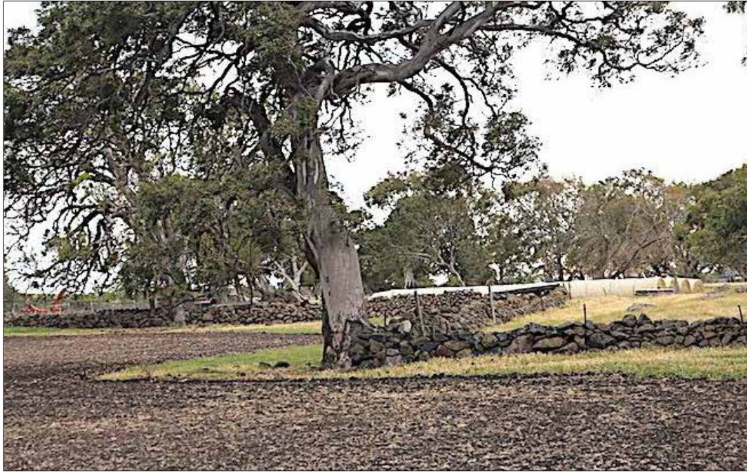
Image 87: Cultivation paddock on CA7, west side of Vearings Road. A stony rise on the right is separated from the arable land by a regularised, stepped, dry stone wall, typical of the Merri–Darebin Plains. (David Moloney, 2019)
