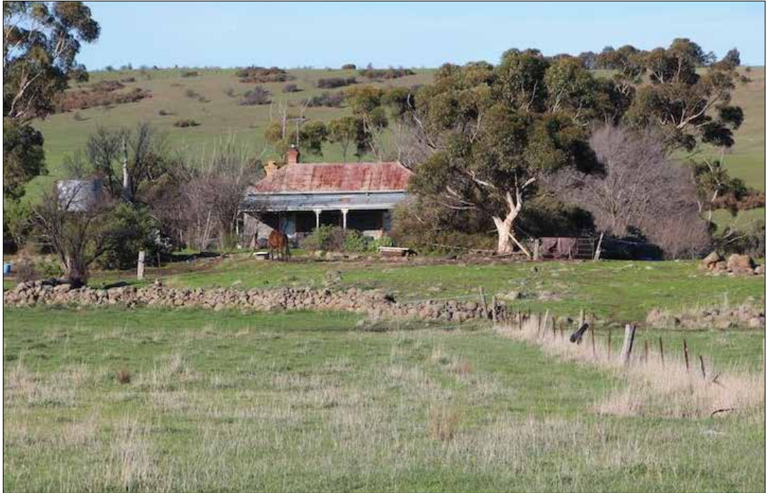
Image 127: 100 Bindts Road, settled by Christian & Maria Bindt in the 1850s. Maria Rosel's family had come to the district via Westgarthtown. The period house is behind a dry stone wall that skirts around a small stony outcrop, and is set in an exceptional rural landscape, with red gums adjacent and Quarry Hill behind. The long north-south stony rise on which it is built features numerous dry stone walls along other Bindts Road properties, in good condition on the ridge, but deteriorating where they move off it. (David Moloney, 2019)
