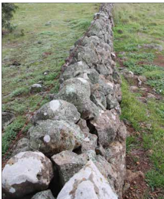
Image 21: The view along the top of the same part of the wall, showing that, despite the use of orthostats wall dimensions are virtually intact, at c.1150 mm high, and c.800 mm at the base, with copestones intact. Sections of this wall have orthostats on both sides. It is not unusual to find intact walls built of orthostats. (David Moloney, 2020)
