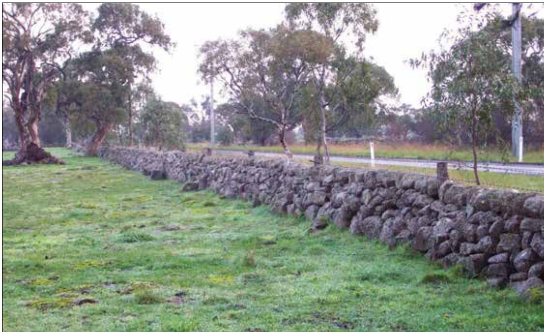
Image 136: Sections of Bindts Road constitute an outstanding and rare example of a double dry stone wall road, the best in the City of Whittlesea. This section is photographed looking north east from the historic Schultz property. Indigenous red gums add to the aesthetic value of the walls. (David Moloney 2019)
