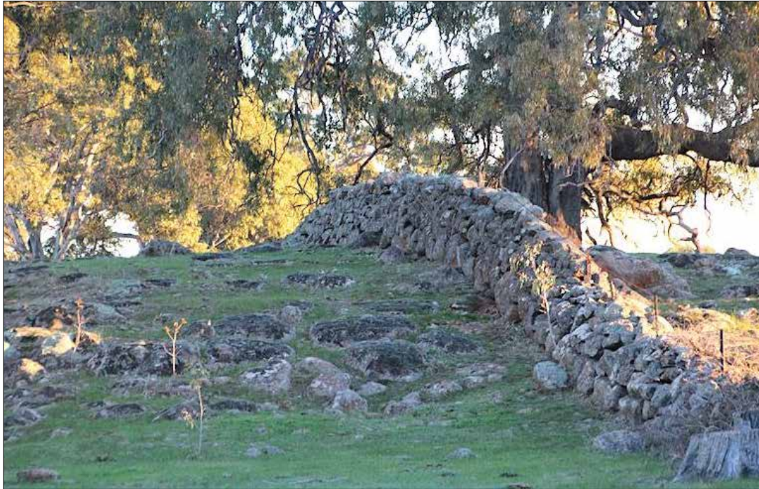
Image 148: 'Fenwick Stud' entrance wall. Being a boundary wall, it forges across instead of around the stony rise and through the red gums, powerfully intact over solid ground. (David Moloney, 2019)
