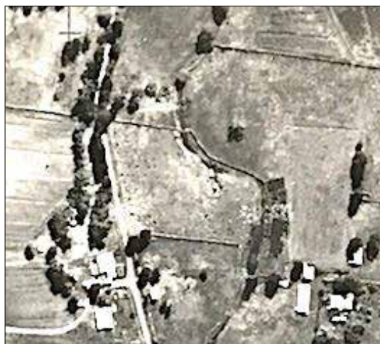
Image 117: Walls converging on and along the creek are visible in this early photograph. The original properties were Heyne and Maltzahn (west) and Winter (east). (Melbourne & Metropolitan Area, 1946)
