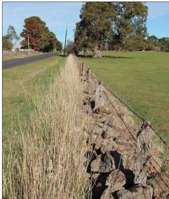
Image 32: Bodycoats Road. Hidden behind the long grass this half-wall features what appears to be uniformly very early posts, with holes drilled for wire at a height commensurate with a half-wall, despite its wide base, which may indicate an original all-stone wall. (David Moloney, 2019)
