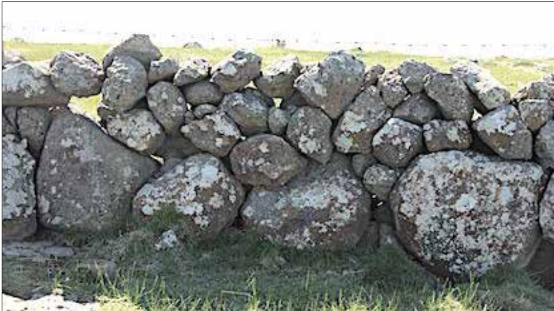
Image 23: Detail of part of the same cultivation paddock wall, showing the oversize foundation stones preventing coursed construction. The foundation stones in this case extend across the whole width of the wall, preventing conventional double-wall construction with hearting, as evident in the light passing through many parts of the wall. (David Moloney, 2019)
