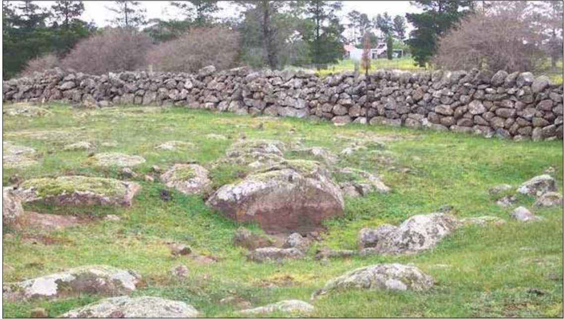
Image 25: This wall (recently demolished) on a stony rise on the original Maryfield on O’Herns Road is also built primarily of angular stone, again with rounder and more uniform-sized stones used as coping. In the foreground is an old quarry or grub-hole, the likely source of some of the stone. (David Moloney, 2000)
