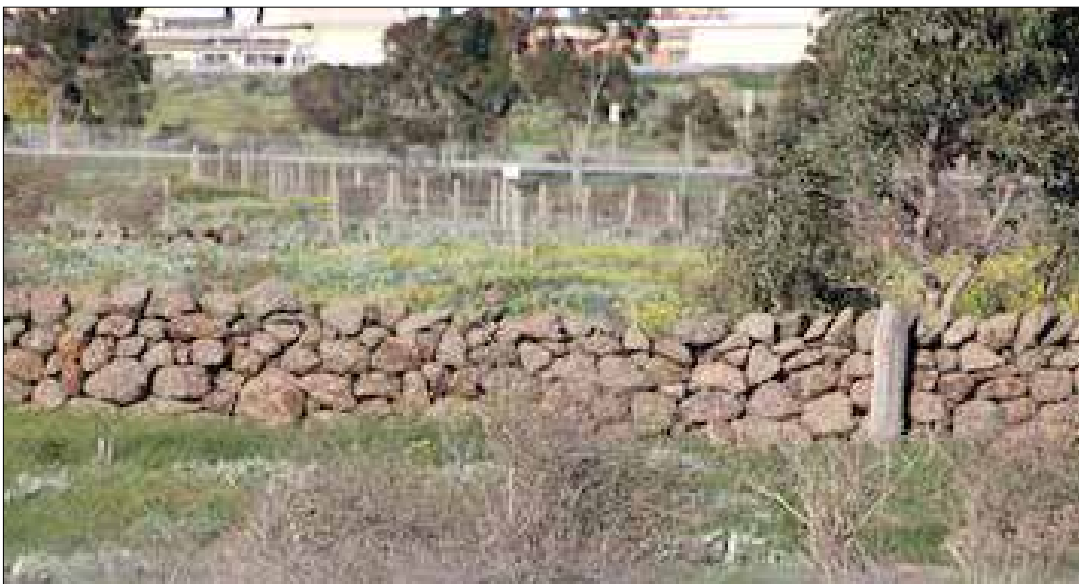
Image 91: Part of the Campbell Estate boundary wall, running north – south, located south of Cooper Street, east of the Epping Wholesale Fruit & Vegetable Market. This part appears to be in good condition, with copestones intact; it appears to be built on a stony rise. (David Moloney, 2019)
