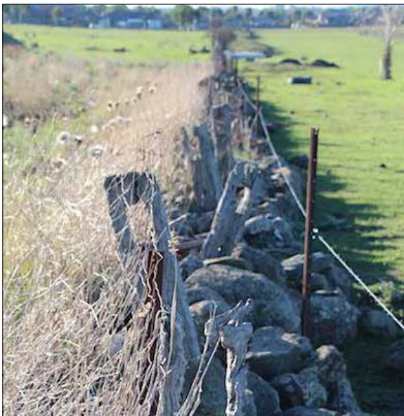
Image 33: This half-wall is the east boundary of a cultivation paddock on the north (Vearings Road) side of O'Herns Road. The uniform height, and (large) uniform sized cope-stones, perhaps on a single-course double base, are indicative of an original half-wall. It contrasts with the double wall along O'Herns Road to which it is perpendicular. The fence posts appear to have been replaced over the course of time; a new post for an electric fence can be seen. (David Moloney, 2019)
