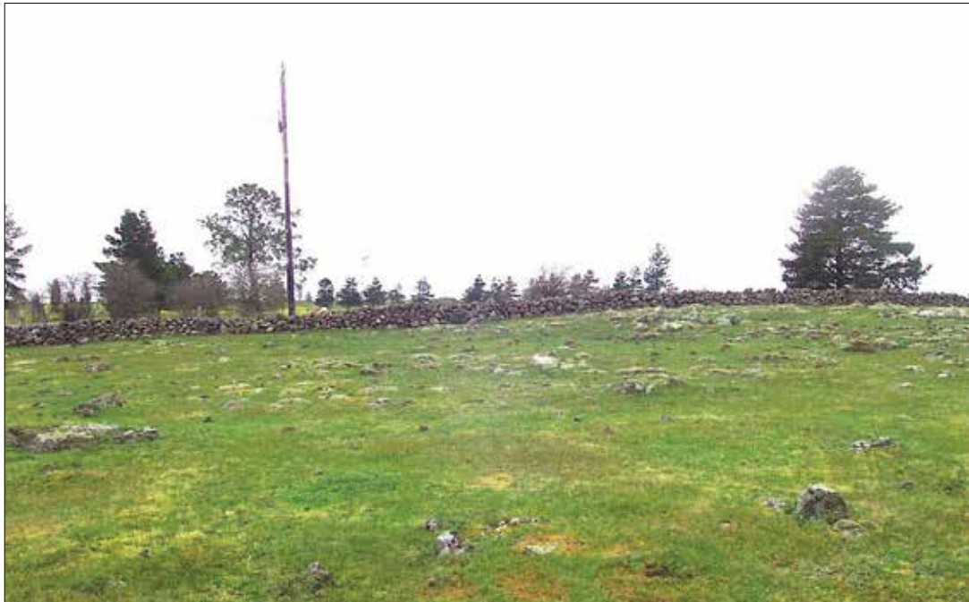
Image 88: Part of the Campbellfield Estate Boundary Wall, O’Herns Road Epping, at near full height as it passed over the stony rise. This wall has only just been demolished. (David Moloney, 2000)
