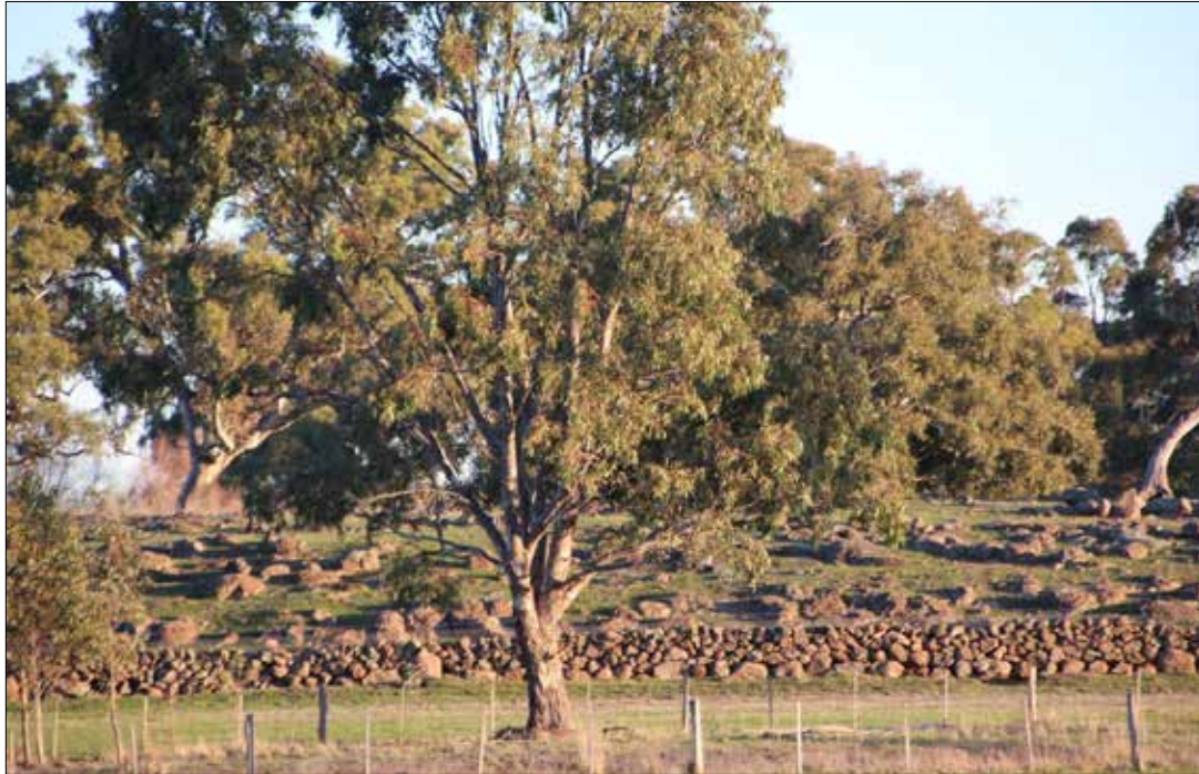
Image 152: Stone wall separating a former cultivation paddock from stony rise on 'Gilghi', immediately west of Fenwick on Donnybrook Road, and of similar setting, scale and style. Like most Whittlesea cultivation paddocks, it features lighter fencing on the softer ground. (David Moloney, 2019)
