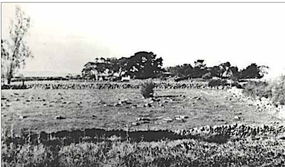
Image 110: Looking east over Nebel’s farm, in the north-east corner of Westgarthtown, c.1910, showing dry stone walls around a stony paddock. The walls appear to be of a more conventional, high and vertical, construction, and to retain most of their original coping. (Photo: per Rob Wuchatsch)
