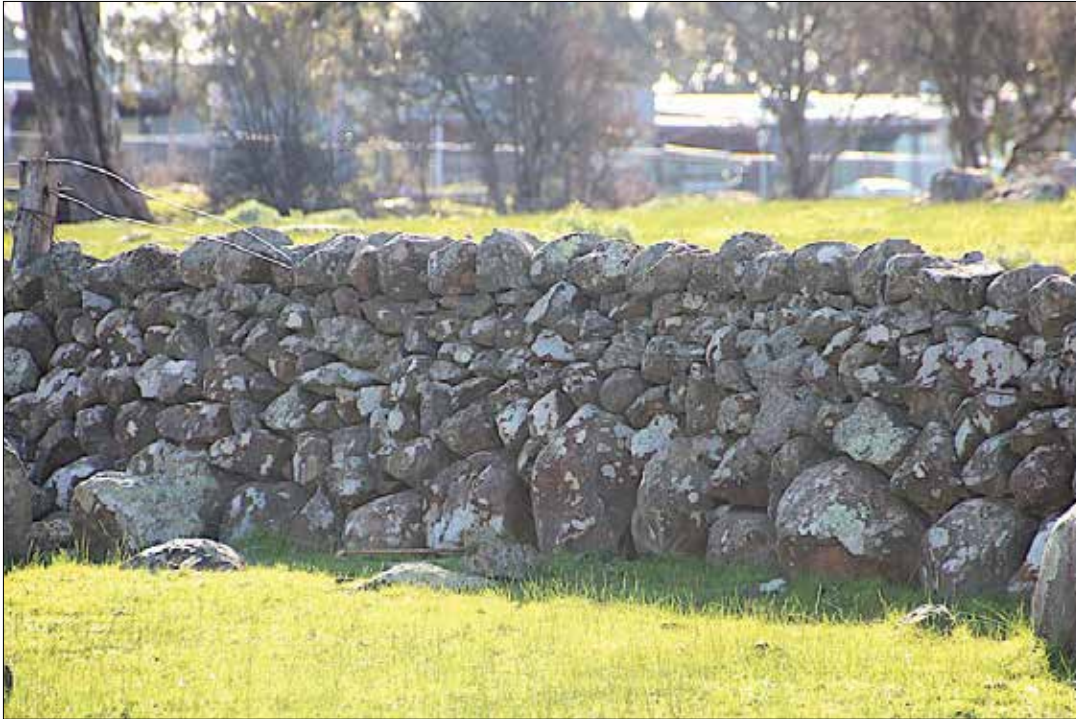
Image 124: 80 Harvest Home Road: at the north end is a regularised or straight cultivation paddock wall, with the stony rise behind. Looking north. (David Moloney, 2019)
