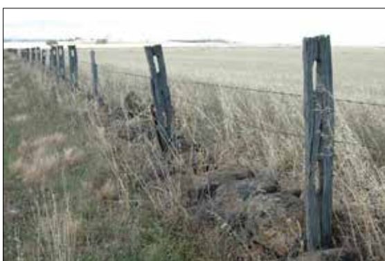
Images 29, 30: Well preserved examples of half-walls in Melton suggest some diagnostics for purpose-built composite walls, including: narrow stone base, sufficient for the intended few courses; consistent construction, regular coping; uniform height; height of the lower hole or mortise; posts and mortises uniform, rather than recycled. Once widespread, purpose-built examples are now relatively few. They may have been built as the result of limited local stone (Peel), and less intensive farming land-uses, for example on the large commercial farms in the south, or the pastoral properties in the north. (David Moloney, 1999)
