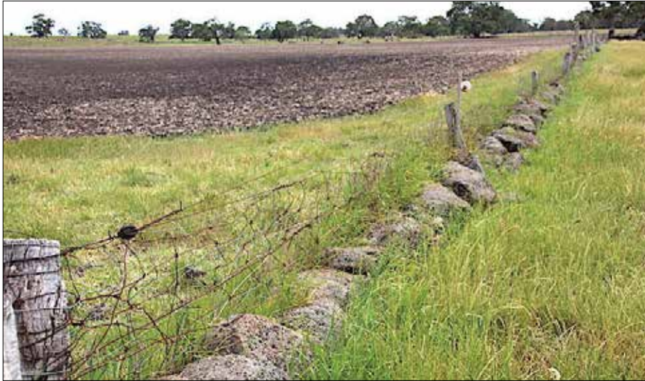
Image 33: This half-wall is the east boundary of a cultivation paddock on the north (Vearings Road) side of O'Herns Road. The uniform height, and (large) uniform sized cope-stones, perhaps on a single-course double base, are indicative of an original half-wall. It contrasts with the double wall along O'Herns Road to which it is perpendicular. The fence posts appear to have been replaced over the course of time; a new post for an electric fence can be seen. (David Moloney, 2019)
