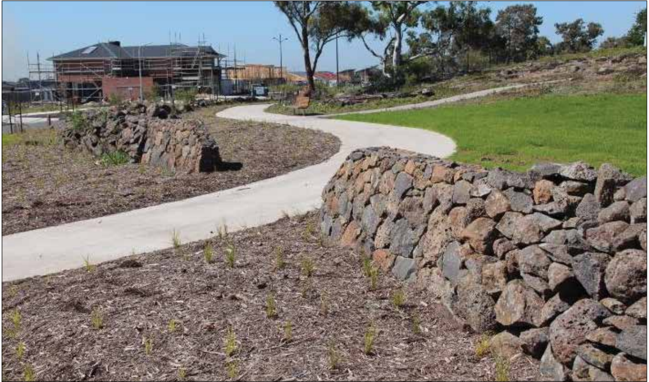
Image 140: Wall face of part of the remarkable stream diversion retaining wall between Lehmanns and Bridge Inn Road, built by Gottlob Ernst Schultz and his sons. The height of this part rises to 1.3 metres. There is a stone apron under the channel in front; the coping stones are at the level of the ground on the other side of the wall. (David Moloney, 2013)
