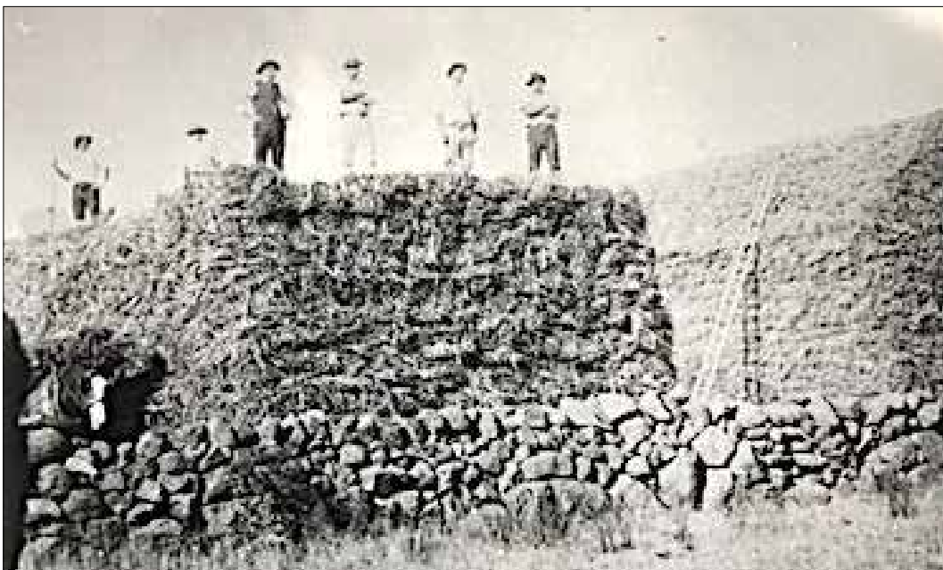
Image 17: Hay Stacking at Schultz's farm, Bridge Inn Road, Wollert (no date), showing oversize foundation stones in wall, rubble construction, with copestones helping tie and secure it. (per Robert Wuchatsch)
