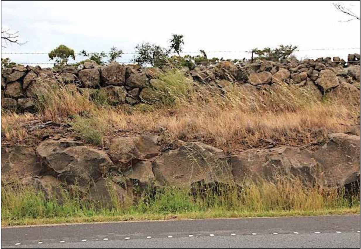
Image 59: No.1220 Donnybrook Road cutting through stony rise, east of Epping Road, south side. Again, showing natural, blocky, fractures in base-rock, and two walls on stony rise in good condition above (one barely visible, behind). (David Moloney, 2019)
