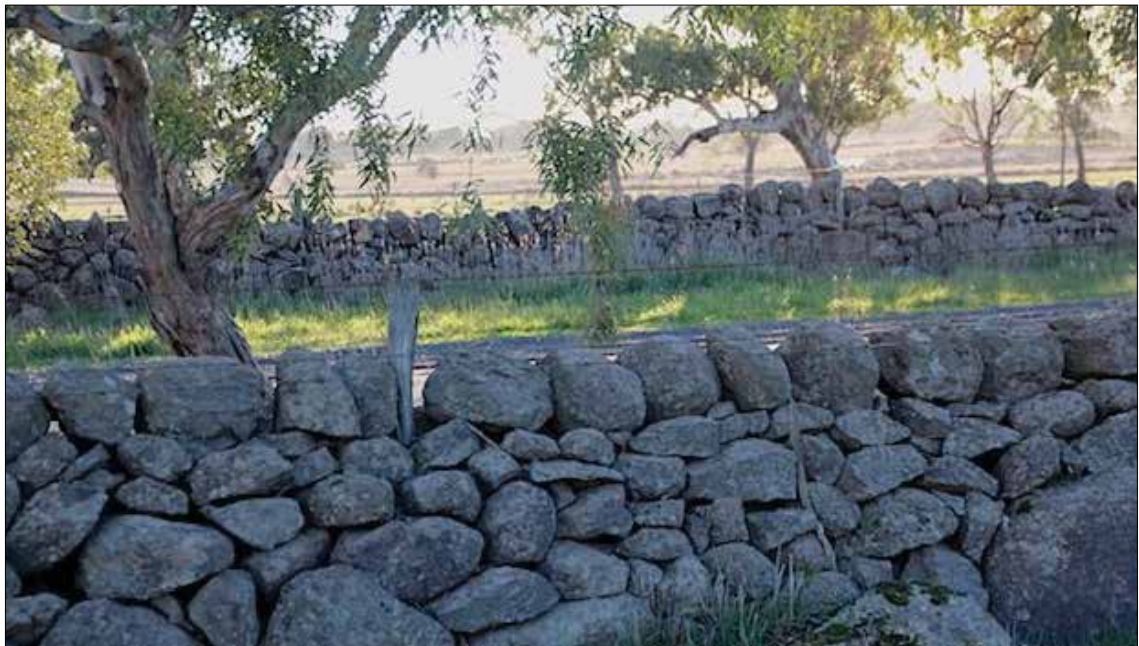
Image 26: This road boundary wall at 240 Bindts Road features large base stones, and also a more equal proportion of rounded and angular stone. A nice array of equally sized and mostly rounded coping stones not only contributes structural stability, but gives a visual cohesion and order to the necessarily random non-coursed construction with the awkward local stones. (David Moloney, 2019)
