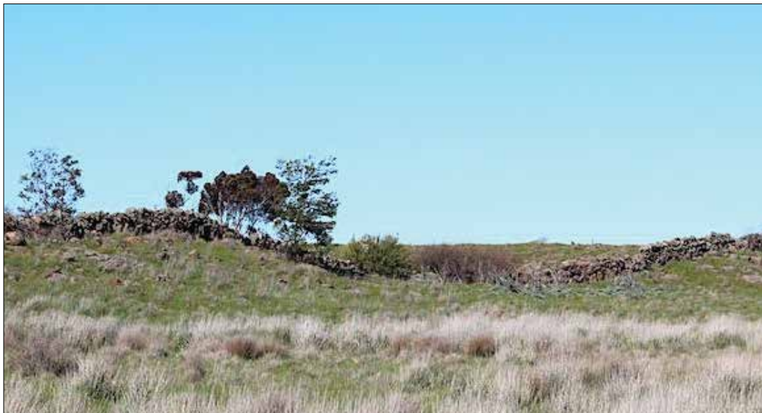
Image 47: A wall marches across the top of stony rises, rather than skirting around them, at 260 Craigieburn Road East. This was clearly a way to build shorter and more durable walls. Also occurring on larger farms in the Western District, this may also reflect reduced pressure to make optimum use of ground available for both pasture and cultivation, as appears to have been the case on the small fresh milk farms in Epping-Wollert. Or it may reflect a different practise, of sometimes allowing grazing on cropped land. (David Moloney, 2019)
