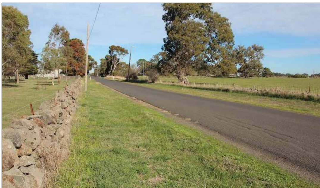
Image 161: Walls on both sides of Bodycoats Road. The left wall is a quite prepossessing repaired all-stone wall. The half-wall on the right, behind uncut grass, is also contributory as a composite stone and post & wire wall. It has very old timbers (some of which nevertheless appear to have been recycled) and may be an original composite, or 'half' wall. However it has a base-width (c.900 mm) which is standard locally, and no evidence of cope-stones, so is apparently an early modification of an original all-stone wall. (David Moloney, 2019)
