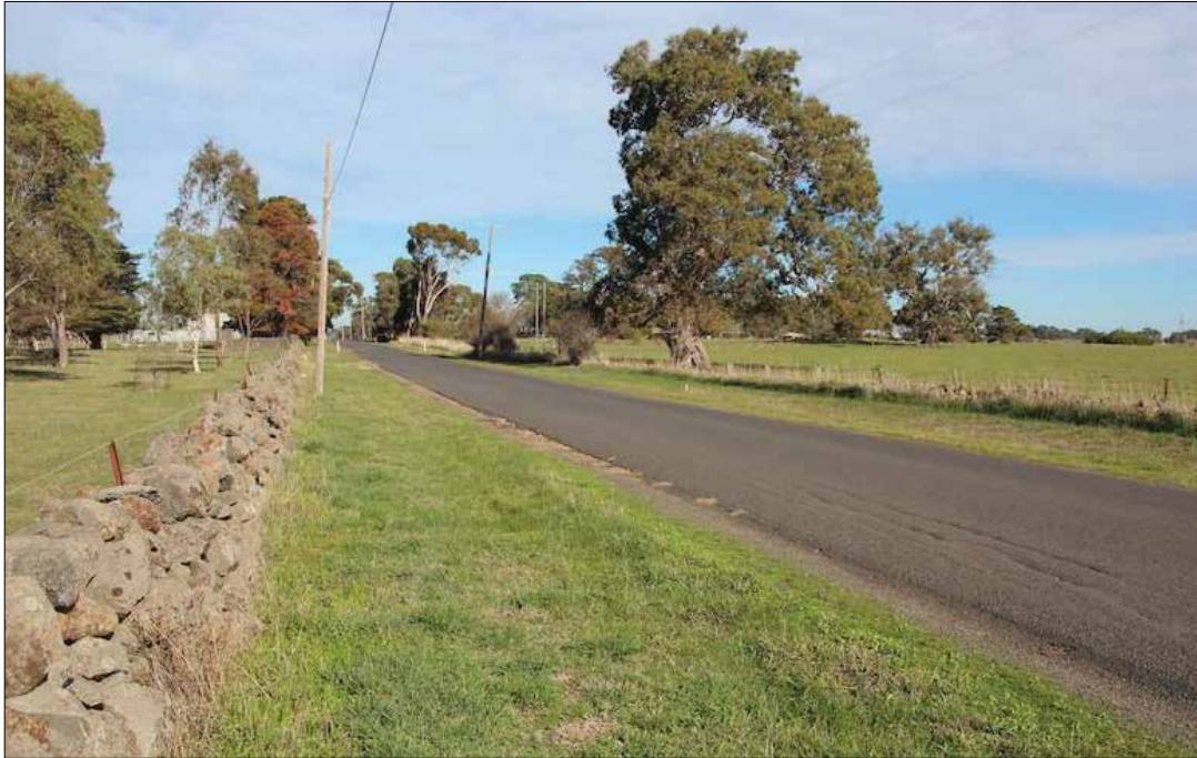
Image 51: Double wall on Bodycoats Road. The left wall is a reasonably prepossessing and well maintained all-stone wall. The half-wall on the right, barely visible behind uncut grass, is also of contributory significance as a characteristic composite stone and post & wire wall. (David Moloney, 2019)
