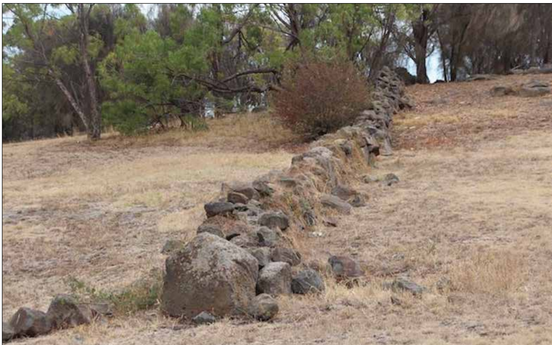
Image 112: East-west dry stone wall on the stony rise south of the church. Many oversize, and some massive stones have been used. (David Moloney, 2019)
