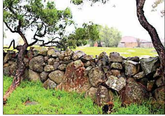
Images 18, 19: The massive or oversize stones in these walls (on the Merri-Darebin Plains, and Westgarthtown Cemetery) govern subsequent construction, which is 'rubble', rather than the 'coursed' orthodox dry stone wall construction system. (David Moloney, 2019, 2012)
