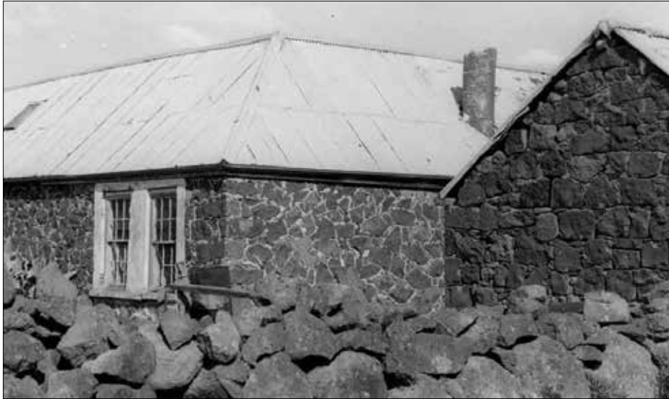
Image 105: Ziebell's Farmhouse and outbuilding before restoration. The rudimentary, oversize and apparently turbulent construction of the Gardenia Road dry stone wall matches the random rubble construction of the residence behind, described by the National Trust as 'almost cyclopean.' 379 (The outbuilding wall by contrast is very roughly coursed.) (State Library of Victoria, Collins, J. (1967). Thomastown [German Town]).
