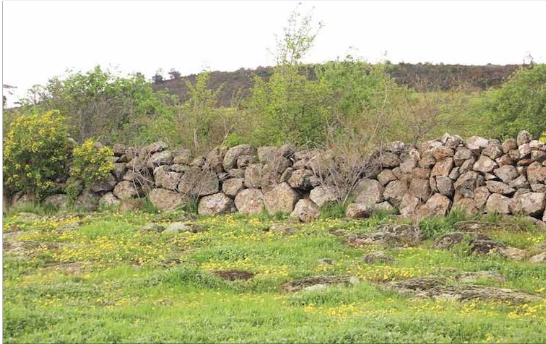
Image 60: The dry stone walled enclosure beside the former Timms house, at 130 Bindts Road Epping. Within the enclosure are a number of very old trees, suggesting a former orchard and perhaps kitchen garden. This part of the enclosure built along the ridge of a stony rise is in good condition. Note the use of oversize and massive stones, some placed on edge, in characteristic Merri–Darebin Plains style. (David Moloney, 2019)
