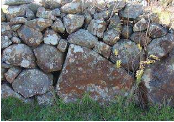
Images 18, 19: The massive or oversize stones in these walls (on the Merri-Darebin Plains, and Westgarthtown Cemetery) govern subsequent construction, which is 'rubble', rather than the 'coursed' orthodox dry stone wall construction system. (David Moloney, 2019, 2012)
