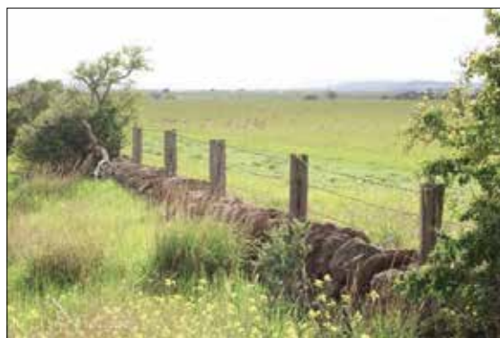
Images 29, 30: Well preserved examples of half-walls in Melton suggest some diagnostics for purpose-built composite walls, including: narrow stone base, sufficient for the intended few courses; consistent construction, regular coping; uniform height; height of the lower hole or mortise; posts and mortises uniform, rather than recycled. Once widespread, purpose-built examples are now relatively few. They may have been built as the result of limited local stone (Peel), and less intensive farming land-uses, for example on the large commercial farms in the south, or the pastoral properties in the north. (David Moloney, 1999)
