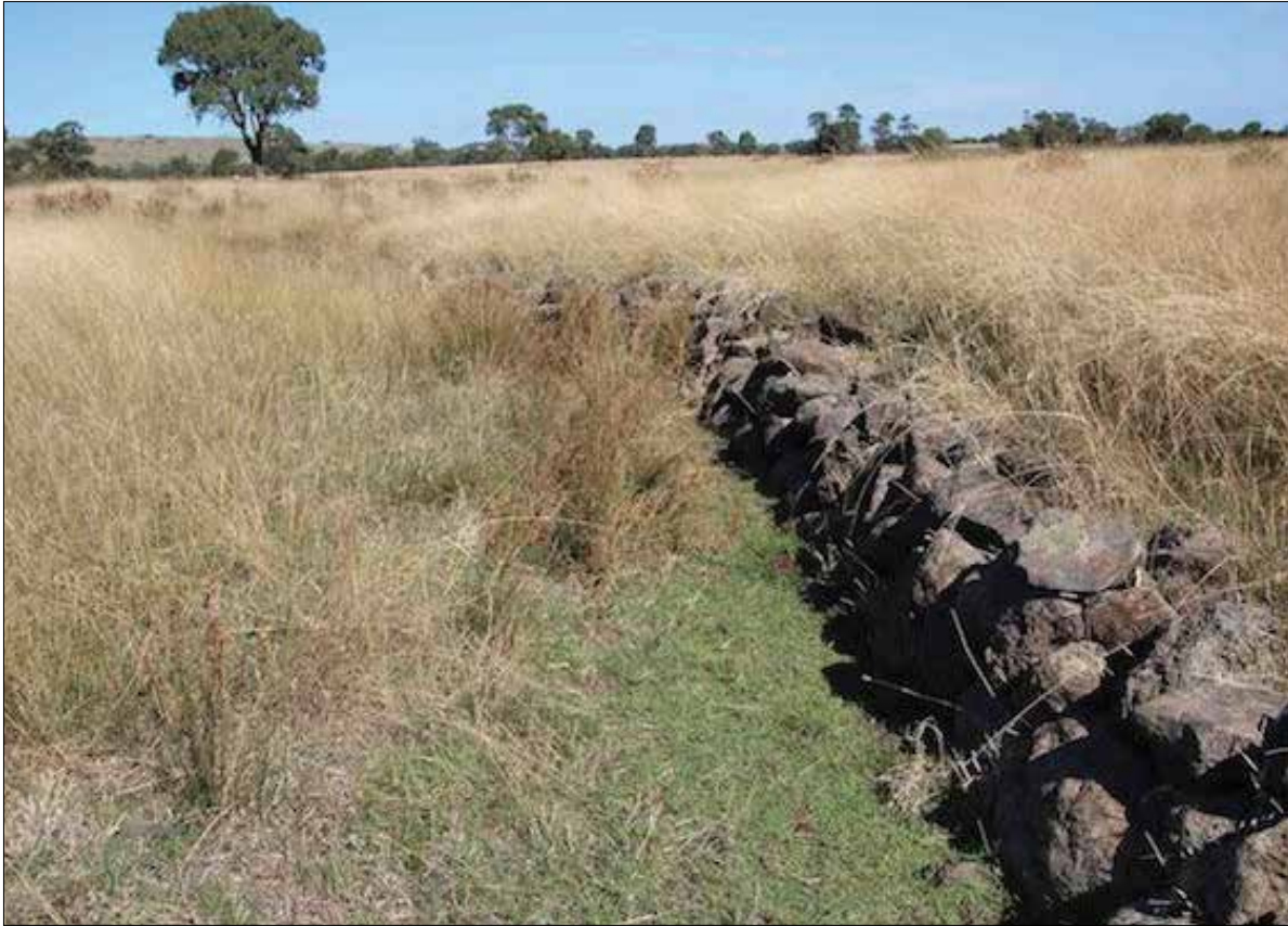
Image 64: Less prepossessing but still substantial, the 'Topp' stream diversion wall, on Schultz property, Lehmanns Road. The west (right) side is just above ground level, and the east (left) side channels the intermittent Findons Creek East Branch. (David Moloney, 2013)
