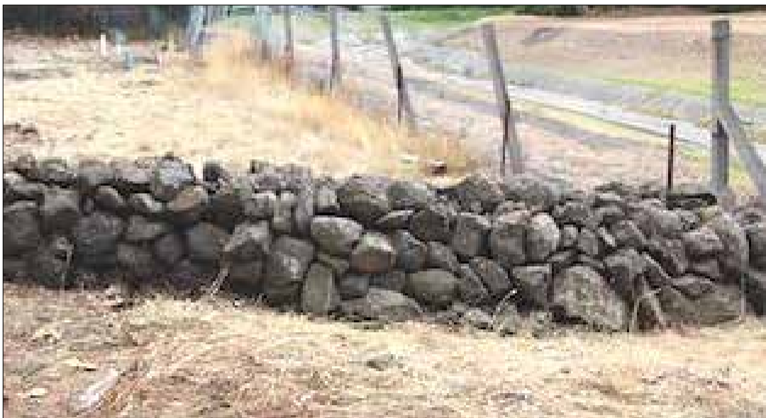
Images 107, 108: Two views of an early wall at the former Wuchatsch homestead, an example of the Westgarthtown 'cyclopean' style, using oversize unworked rounded stones, with minimal vesicularity, held together by their weight, and judicious placement of smaller stones. While large, these stones are fairly uniform in size, without more massive stones intruding, which enables a semblance of coursing. The wall is typical of Westgarthtown walls in terms of its large stone.
