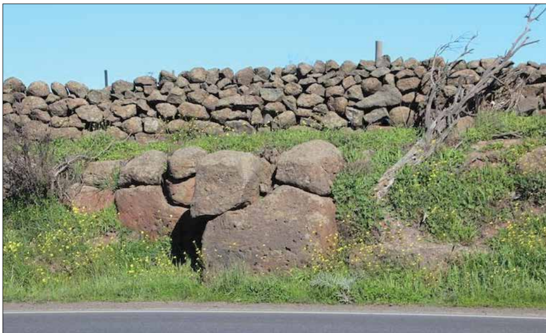
Image 58: Craigieburn Road East, south side, cutting through a stony rise, provides a very prominent example of an intact section of dry stone wall on top of the stony rise; the wall collapses across lower ground immediately to the east. Note the blocky fractures in the base rock. (David Moloney, 2019)
