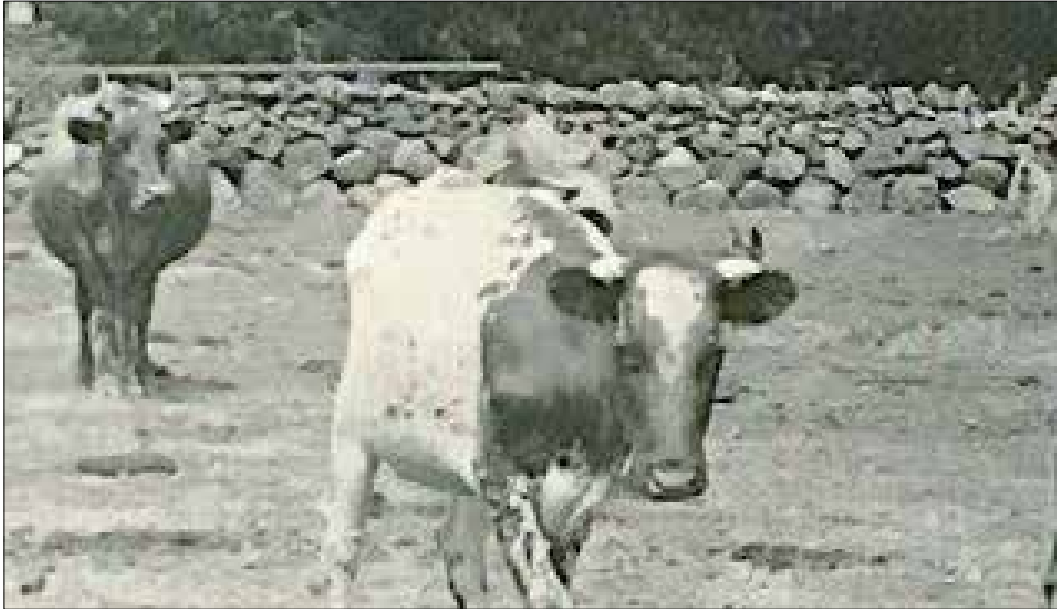
Image 16: Historical photograph showing a typical style of wall, on the John Wuchatsch (junior) farm at O'Herns Road Epping. The wall has some very large stones, although fewer than those on Gardenia Road Westgarthtown, and perhaps less massive. It also has a more equal proportion of rounded and angular stone, with regular sized rounded cope stones. (per Robert Wuchatsch)
