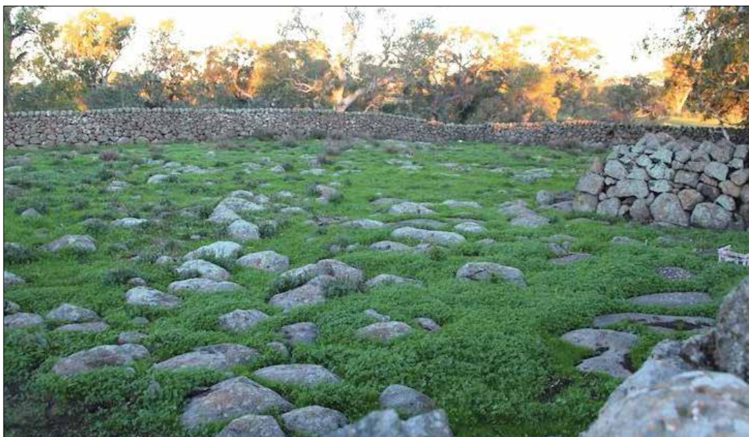
Image 61: Fenwick Stud horse yard on Donnybrook Road encloses an extremely large area. Some of its walling is over two metres high, and appears to be professionally built. A portion has recently collapsed and needs repair. (David Moloney, 2019)
