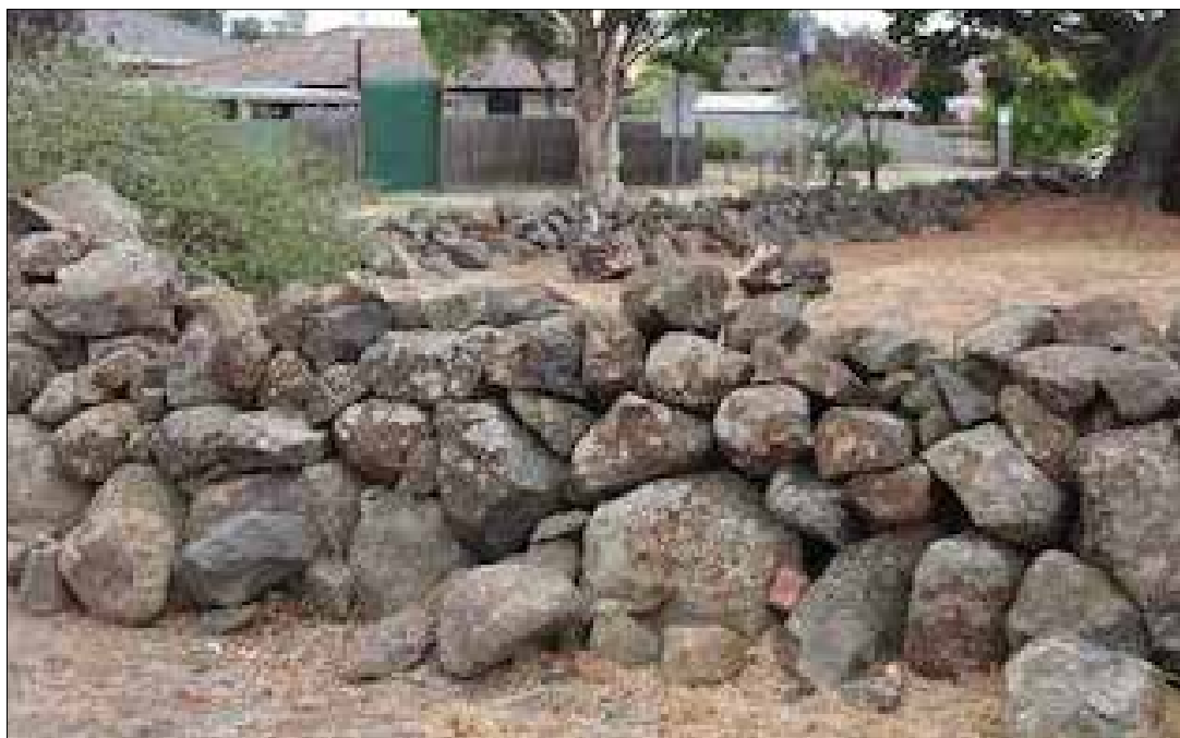
Image 114: The same corner of the cemetery today, with missing upper courses and copestones. (David Moloney, 2019)
