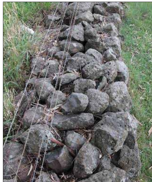
Images 55, 56: Bridge Inn Road. A conventional 'double wall', which is strikingly and typically more intact where it passes over a stony rise. The section at left is close to its original condition, with a base of 800 mm, and height of 900 mm – 1250 mm. The majority of the same wall on softer ground (right) has spread to be c.1300 mm wide at the base, and is only c.550 mm high. (David Moloney, 2013)
