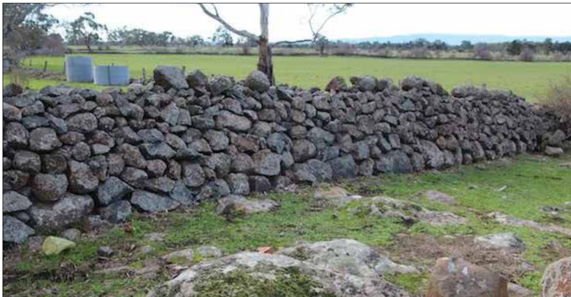
Image 24: Milking yard wall on a stony rise on the former William Bodycoat farm. While in this case there are no massive or oversize stones, the wall demonstrates the high proportion of angular stone in typical Whittlesea walls. Nearby are a number of small quarries on rocky outcrops, the likely source of some of this stone. As is typical, the rounder stones, mostly fieldstone gathered from the surfaces of the knolls or paddocks, are used as the coping, although most are now missing here. The small loose boulders in the foreground appear to have been common on local stony rises. (David Moloney, 2019)
