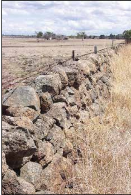
Image 57: Typically intact and short (c.30 metres) section of a road wall over a stony rise, O'Herns Road. (David Moloney, 2009)
