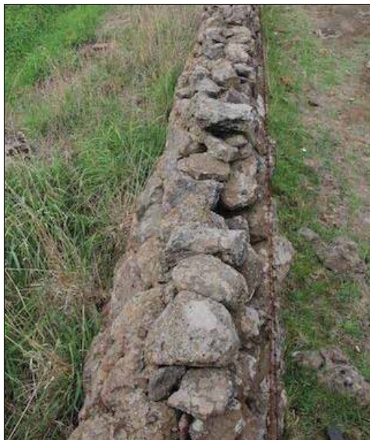
Images 55, 56: Bridge Inn Road. A conventional 'double wall', which is strikingly and typically more intact where it passes over a stony rise. The section at left is close to its original condition, with a base of 800 mm, and height of 900 mm – 1250 mm. The majority of the same wall on softer ground (right) has spread to be c.1300 mm wide at the base, and is only c.550 mm high. (David Moloney, 2013)
