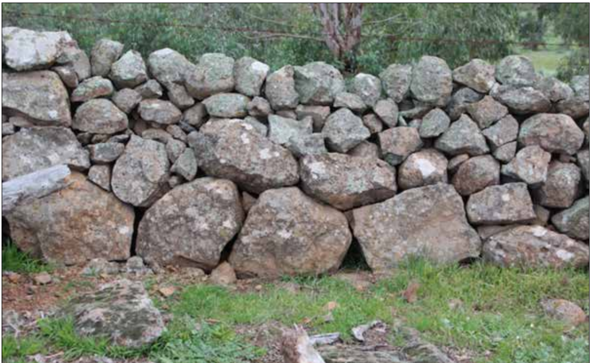
Image 20: Orthostats on the bottom course of a stony rise boundary wall between Fenwick Stud and the Growling Frog Golf Course, Donnybrook Road. That these are stones placed on edge rather than boulders is evident from the flattish faces of the stones. (David Moloney, 2020)
