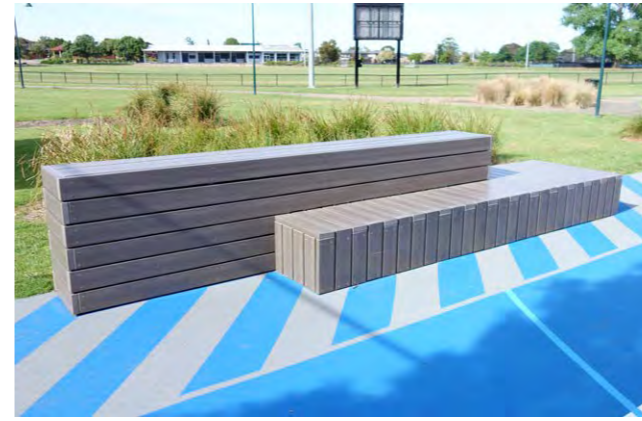
1.9 Tiered seating constructed with wood plastic composite
