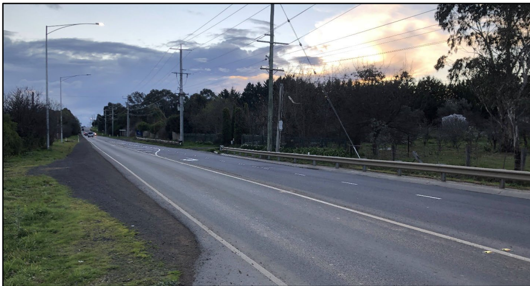
Figure 4 Bridge Inn Road – facing west
