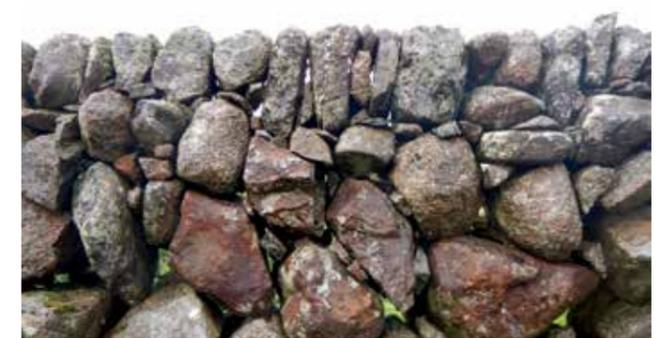
**Figure 8** Construction Style – Single wall.
