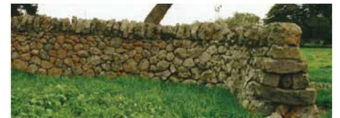
**Figure 9** Construction Style – Double wall. The wall end at right, shows the wall's cross-section detail.
