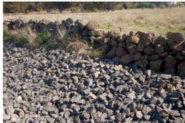
**Figure 34** Subjective Repair Quality – Poor. A rubble wall (right) has been reinstated to join a Galloway style wall (left). The Galloway wall is in fair condition. The stone fill in the foreground is recent and placed in the roadside "gutter."
