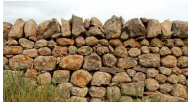
**Figure 17** Stone Shape – Rounded.
