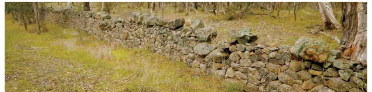
**Figure 32** Subjective Condition – Good. The wall has many minor gaps but full-height wall remains.
