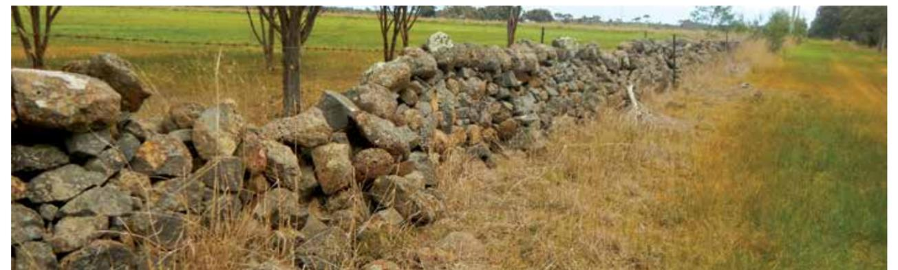
**Figure 33** Subjective Condition – Fair. This wall has surviving characteristics to identify it as a double wall with coping but height is variable due to collapse and slumping. Fallen stone has been crudely returned to the gaps.
