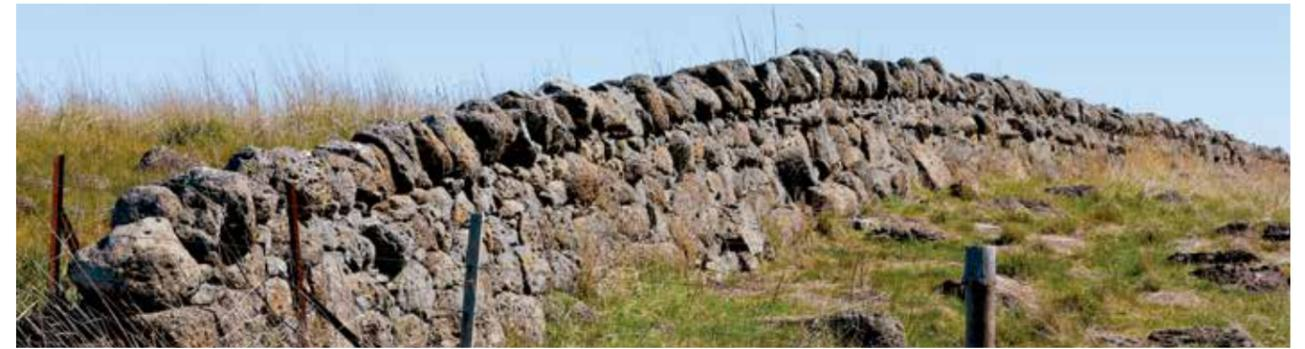
**Figure 30** Subjective Condition – Excellent. A length of wall in original condition for line, height, style with no missing stone. Note the line of projecting throughstones.
