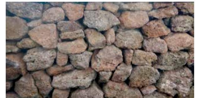
**Figure 23** Stone Surface – Vesicular, with naturally occurring holes.
