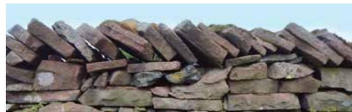
**Figure 27** Coping Pattern – Inclined.
