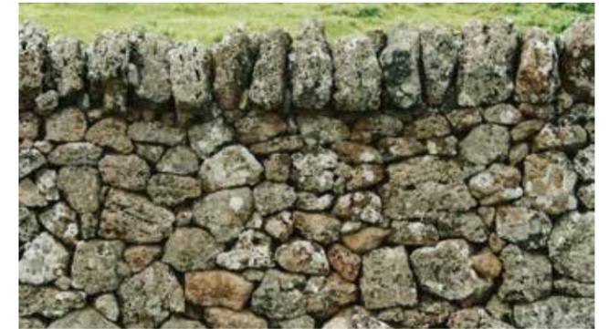
**Figure 14** Stone Size – Common. Stone is of a size which is easily lifted and placed in the wall.
