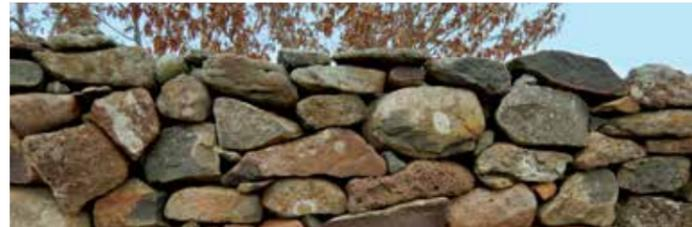
**Figure 24** Coping Pattern – None. Figure shows wall levelled to height with small stones but not described as cope stones.
