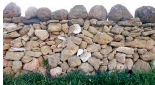
**Figure 13** Stone Type – Limestone. The copestones are vesiculated basalt.
