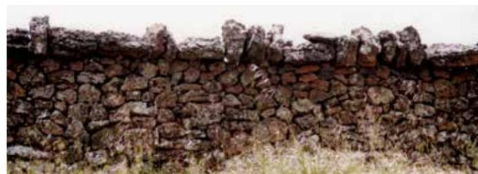
**Figure 28** Coping Pattern – Cock and Hen. Multiple uprights and flats are repeated to form the pattern.
