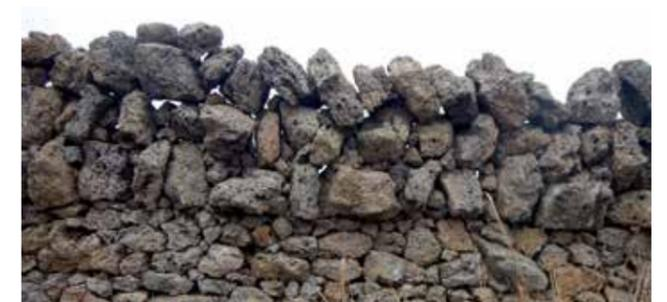
**Figure 10** Construction Style – Galloway wall. This example built with highly vesiculated basalt stone. Vesiculated basalt – having visible surface holes or cavities in the rock.
