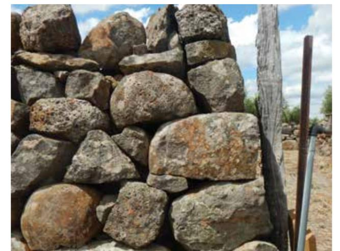
**Figure 16** Stone Size – Oversized. Figure shows a wall end and section of face.
