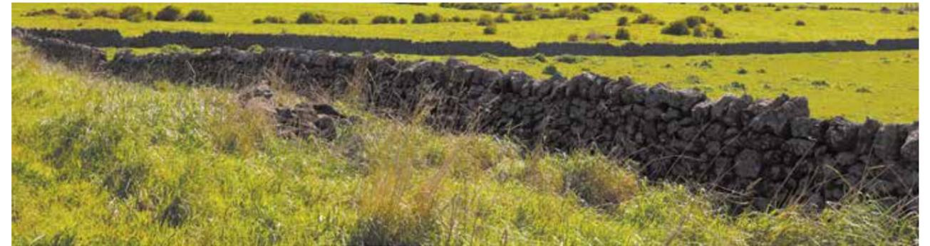
**Figure 31** Subjective Condition – Very Good. Two wall sections in substantially original condition downgraded due to the isolated gaps and missing coping stone.
