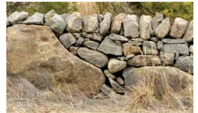
**Figure 15** Stone Size – Cyclopean common-sized stones complete the upper portion of the wall.
