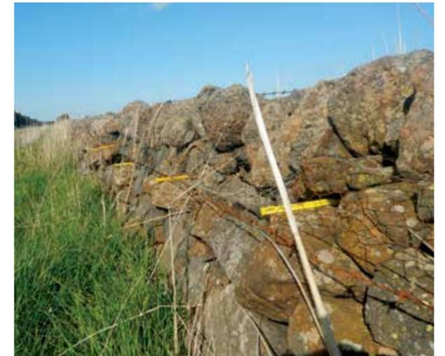
**Figure 29** Throughstone Placement – Projecting. Yellow pegs have been placed to highlight each projecting throughstone.
