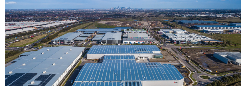
4Ten, Cooper Street West and South West Employment Precinct, Epping.
