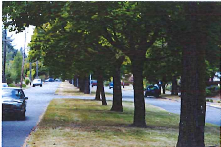
Road reserve can accommodate large plantings to increase the sites overall amenity, create visual interest & to form organizing elements to key points of interest
