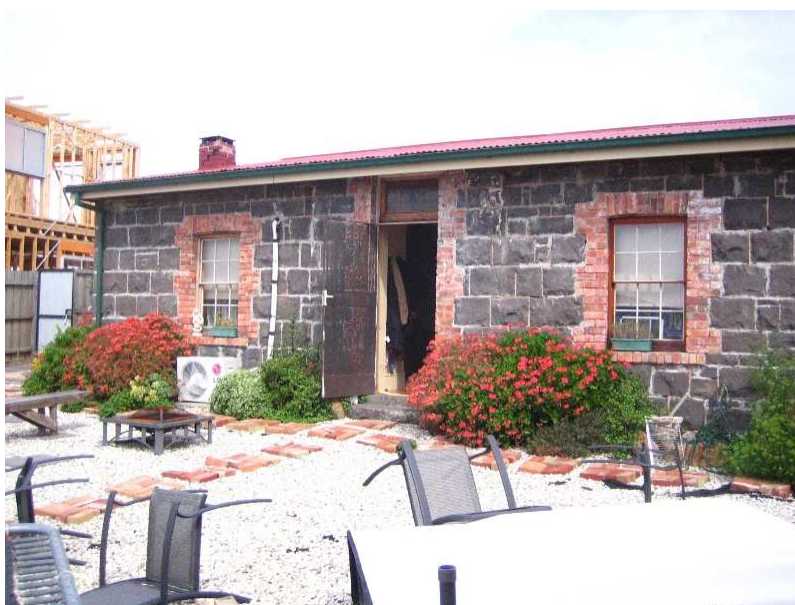
1 Cottage Boulevard, original front facade
