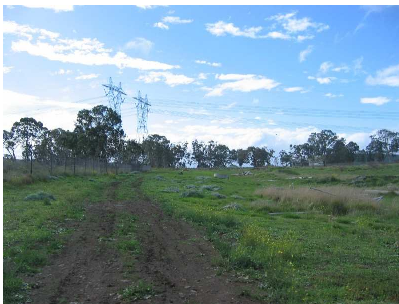
YAN YEAN PIPETRACK (DANAHER DRIVE)
