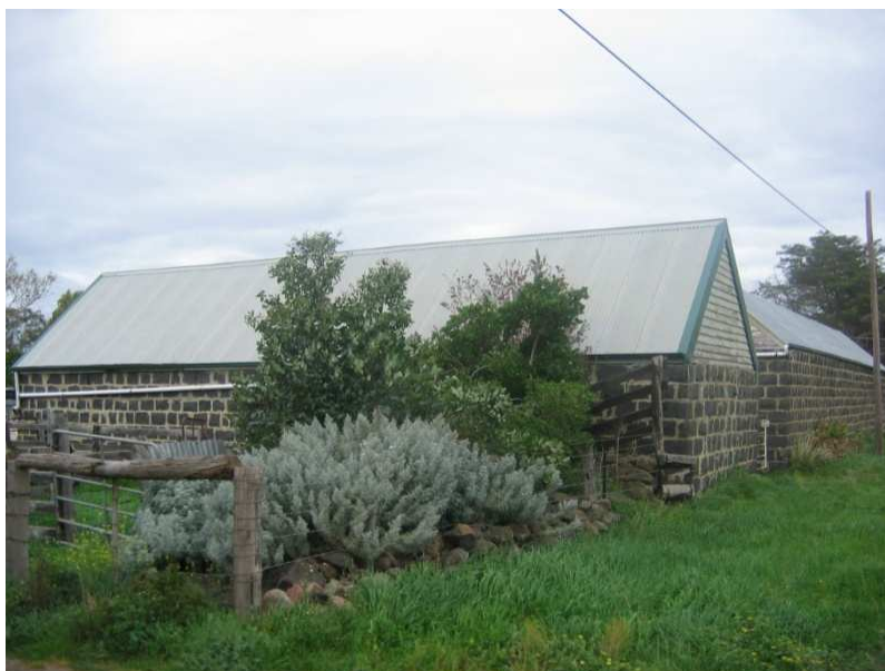
Springvale-Bodycoats Farm, bluestone barn and milking shed
