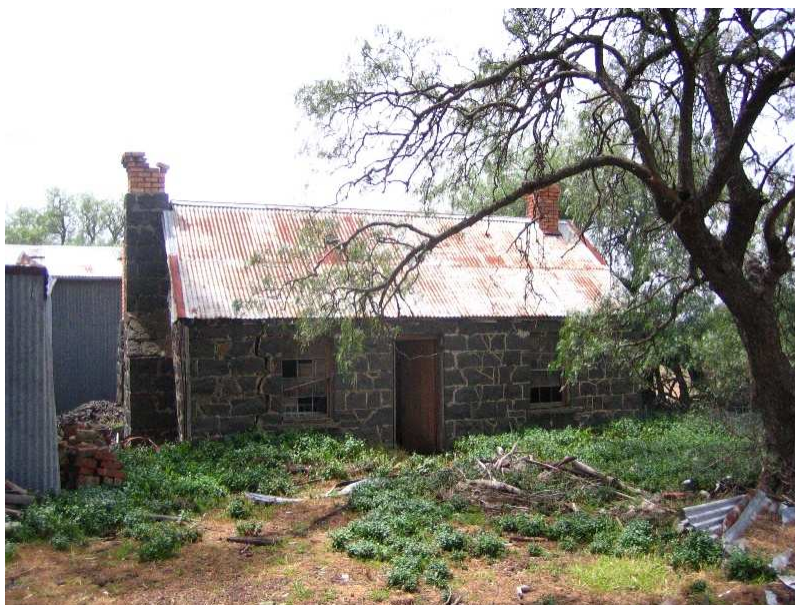
700 Epping Road, bluestone (Stimsons) house
