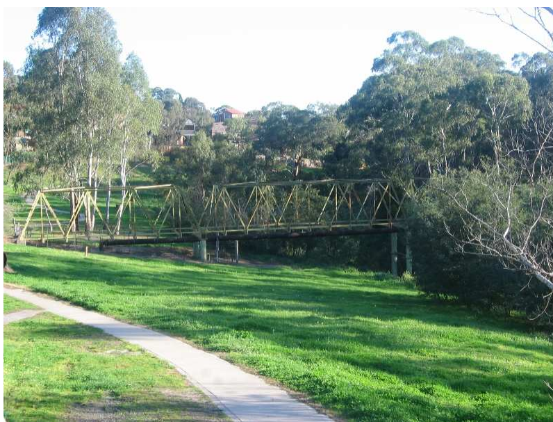
Maroondah Aqueduct Bridge
