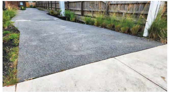
Figure 31 Permeable concrete driveway in Ringwood
