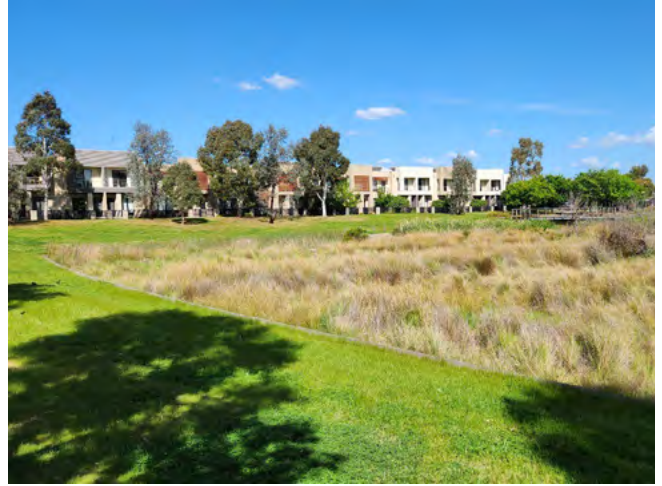
Figure 43 Large-scale biofiltration system at Moffat Park, Lalor
