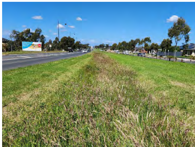
Figure 49 Vegetated swale along Craigieburn Road East, Wollert
