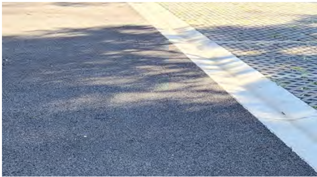
Figure 29 Open graded asphalt wearing course on School Road car park, Menzies Creek
