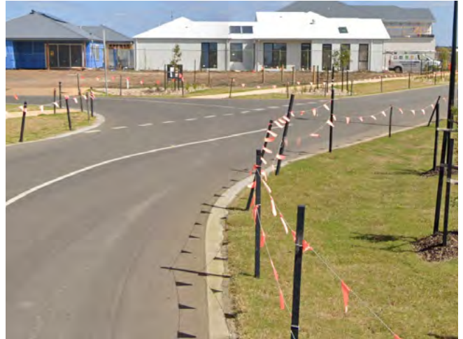
Figure 50 Mowable swale with concrete edge strip on Chiton Way, Point Lonsdale
