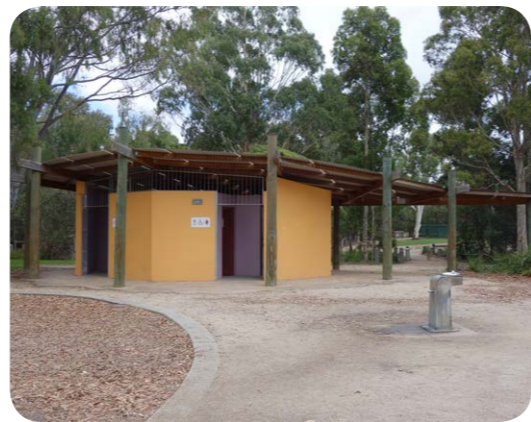
1.4 Existing Toilet Facility - Roof to be retained
