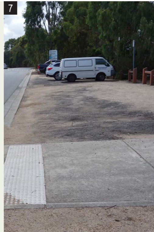
90° car parking with granitic sand surfacing
