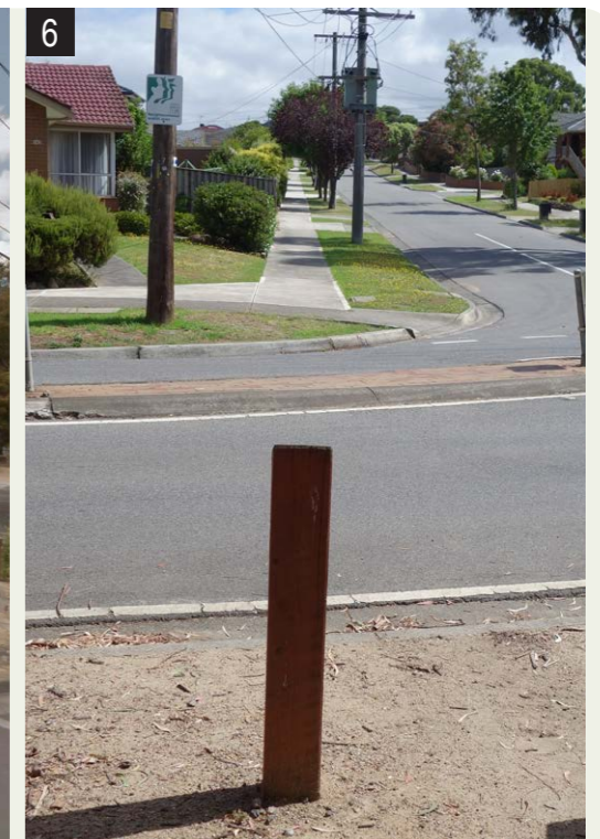
6 Disconnected and inaccessible entry point
