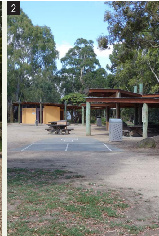
2 Existing picnic area and public toilet
