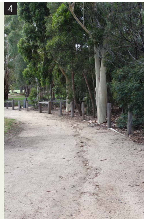
4 Granitic sand path condition
