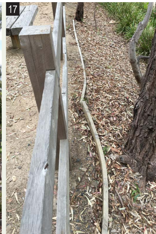
Timber edging, fence and bench
