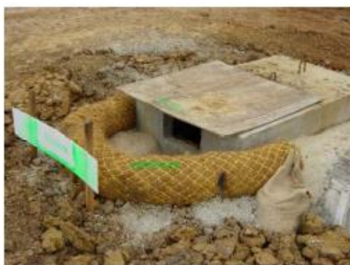
Coir Log utilised for inlet protection (EPA Publication 960)
