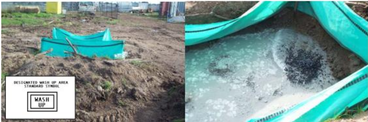
Designated Concrete Washout Area
