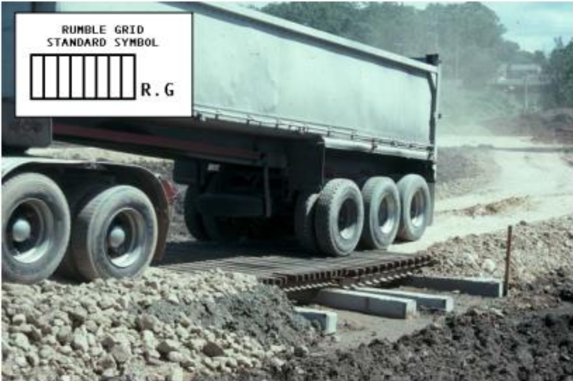
Stabilised Access Point / Rumble Grid (EPA Publication 960)
