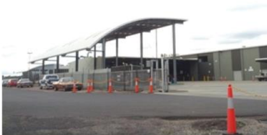
2. Dyson Bus Company Sheds
