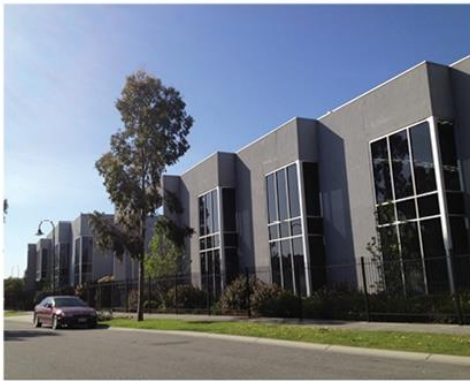
1. Good quality two storey built form
