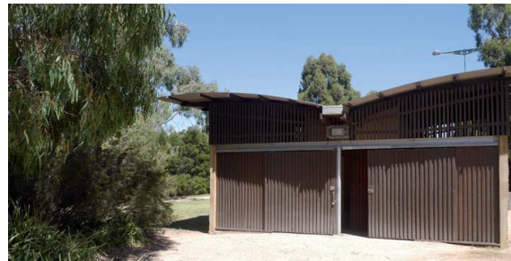
Photo 14: Existing Toilet block
