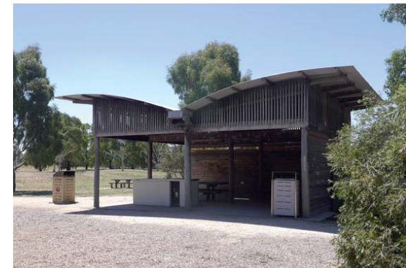
Photo 15: Existing Picnic Shelter and BBQ
