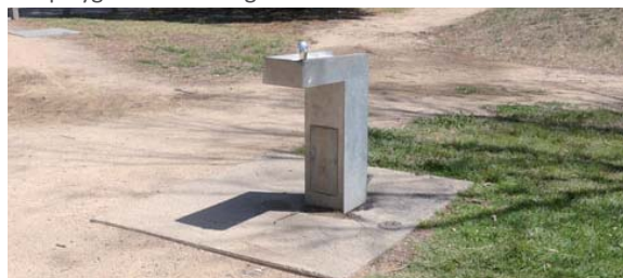
Photo 18: Existing Drinking Fountain
