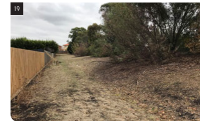
Open grassed drainage swale along southern boundary
