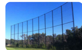
Example of ball protection fence
