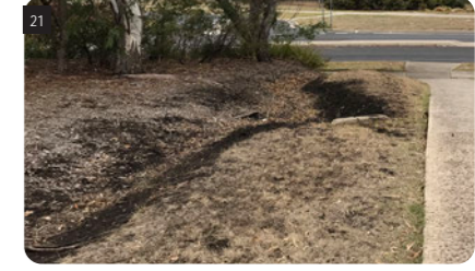
End of open drainage swale
