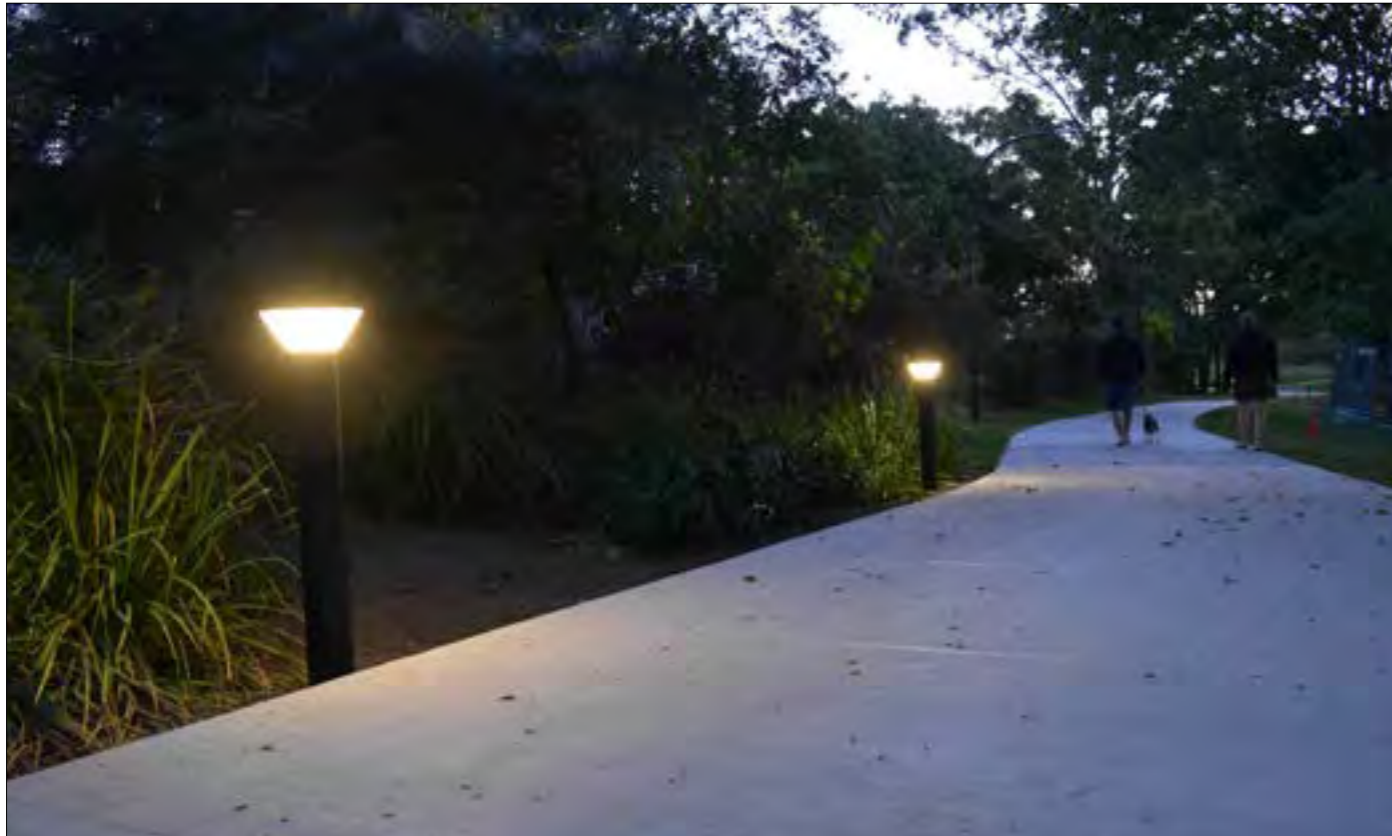
5B. Example of bollard solar lighting
