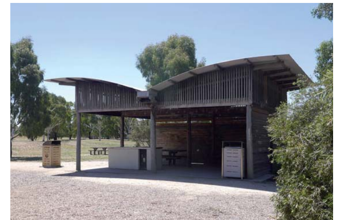
Photo 15: Existing Picnic Shelter and BBQ
