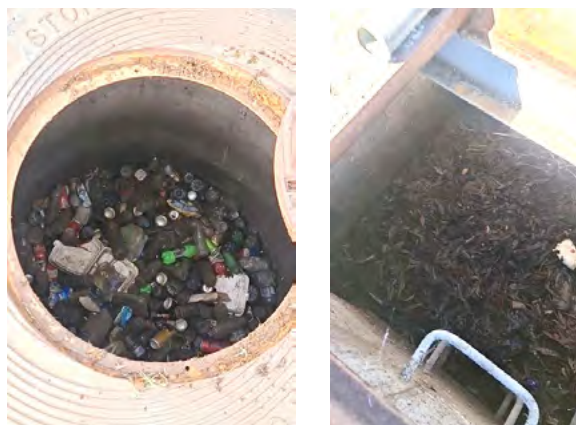
Figure 52 Gross pollutant capture in proprietary products
