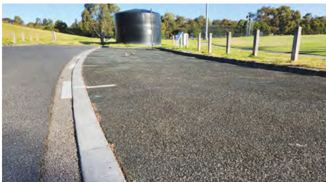
Figure 30 Permeable tyre-derived aggregate wearing course on Ramsden Street, Clifton Hill
