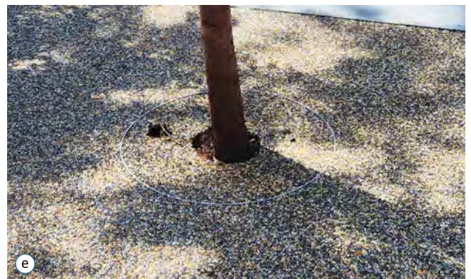
Figure 21 Passively irrigated urban trees: a) and b) side entry pit bypass for catchment increase (Fernhill Road, Mt Evelyn), c) interlocking block pavers and mulch combination (Were Street, Montmorency), d) pervious tyre-derived aggregate (TDA) pavement used around existing tree (Were Street, Montmorency), e) planting in permeable resin-bound aggregate with sacrificial steel ring (Hume Civic Centre, Broadmeadows)
