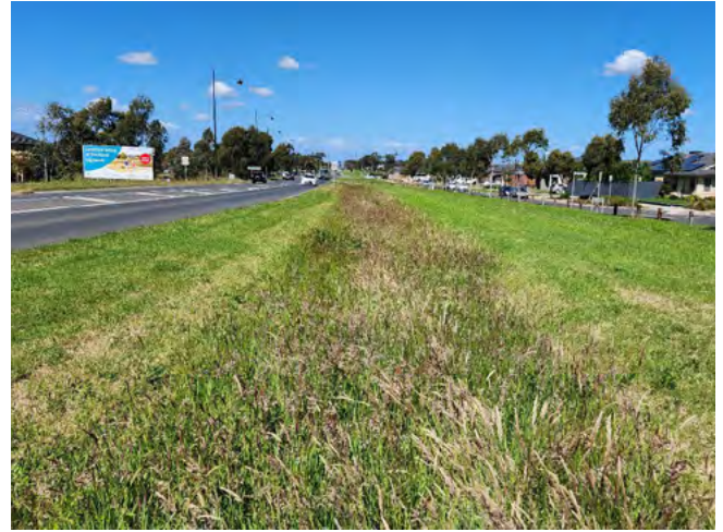
Figure 49 Vegetated swale along Craigieburn Road East, Wollert
