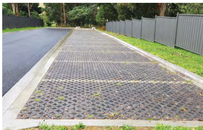
Figure 33 Concrete grid pavement with screenings infill on School Road car park, Menzies Creek
