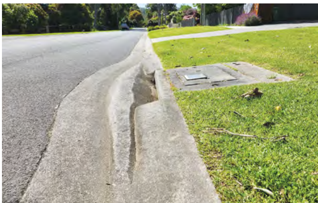
Figure 44 Side entry pit low-flow bypass in Fernhill Road, Mount Evelyn
