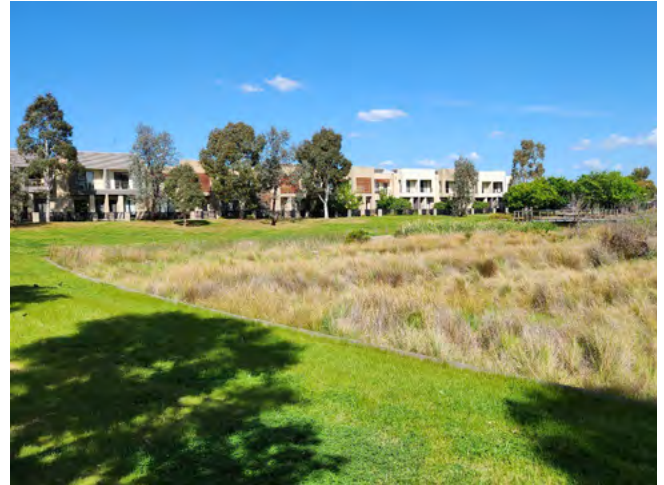
Figure 43 Large-scale biofiltration system at Moffat Park, Lalor
