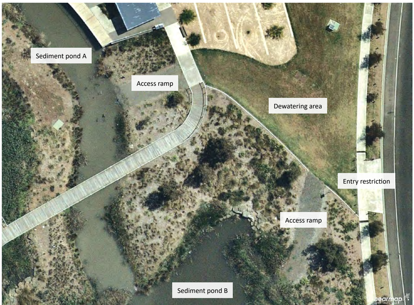
Figure 42 Access, ramping and sediment dewatering provisions at sediment ponds
