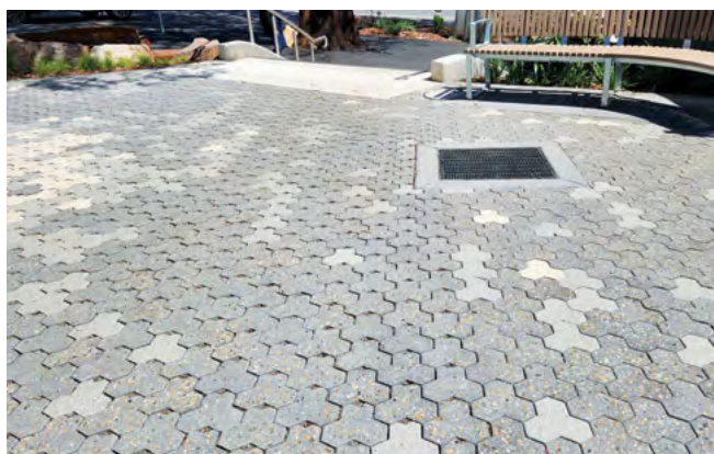
Figure 32 Permeable interlocking concrete pavers (modified tri-hex) adopted on Were Street, Montmorency
