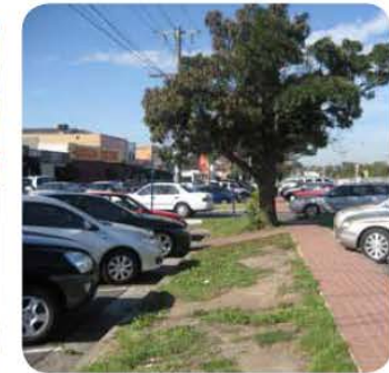
Poorly maintained carpark landscape buffer areas
