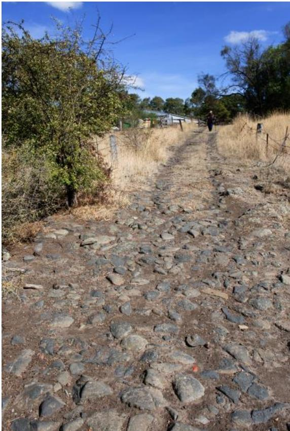
Figure 7. Rubble stone paved track leading from milking shed to Darebin Creek 2019
